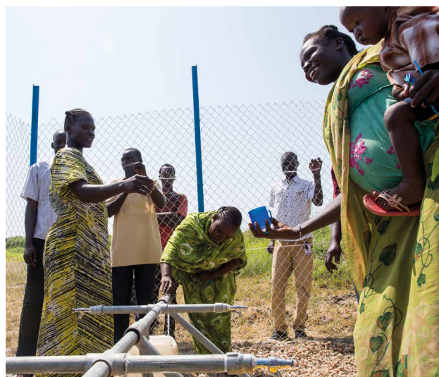
Solar-powered mini wateryard facility in Gormoyok Village in Juba County, Central Equatoria State. Photo credit: UN Photo/JC McIlwaine
