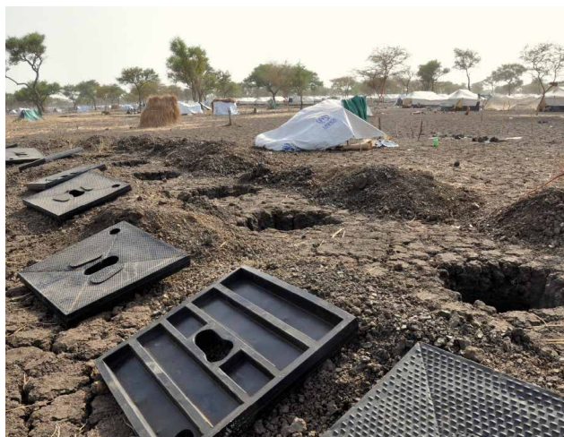
Latrine slabs waiting to be installed, Jamam refugee camp. Photo credit: Oxfam International/Flickr.com/CC BY-NC-ND 2.0
