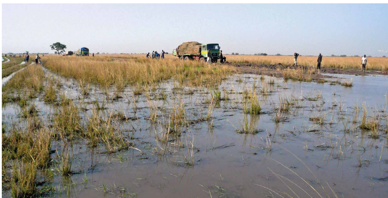
Poor road network: road between Thiet and Tonj. Photo credit: Steffen Emrich/Flickr.com/CC BY-ND 2.0
