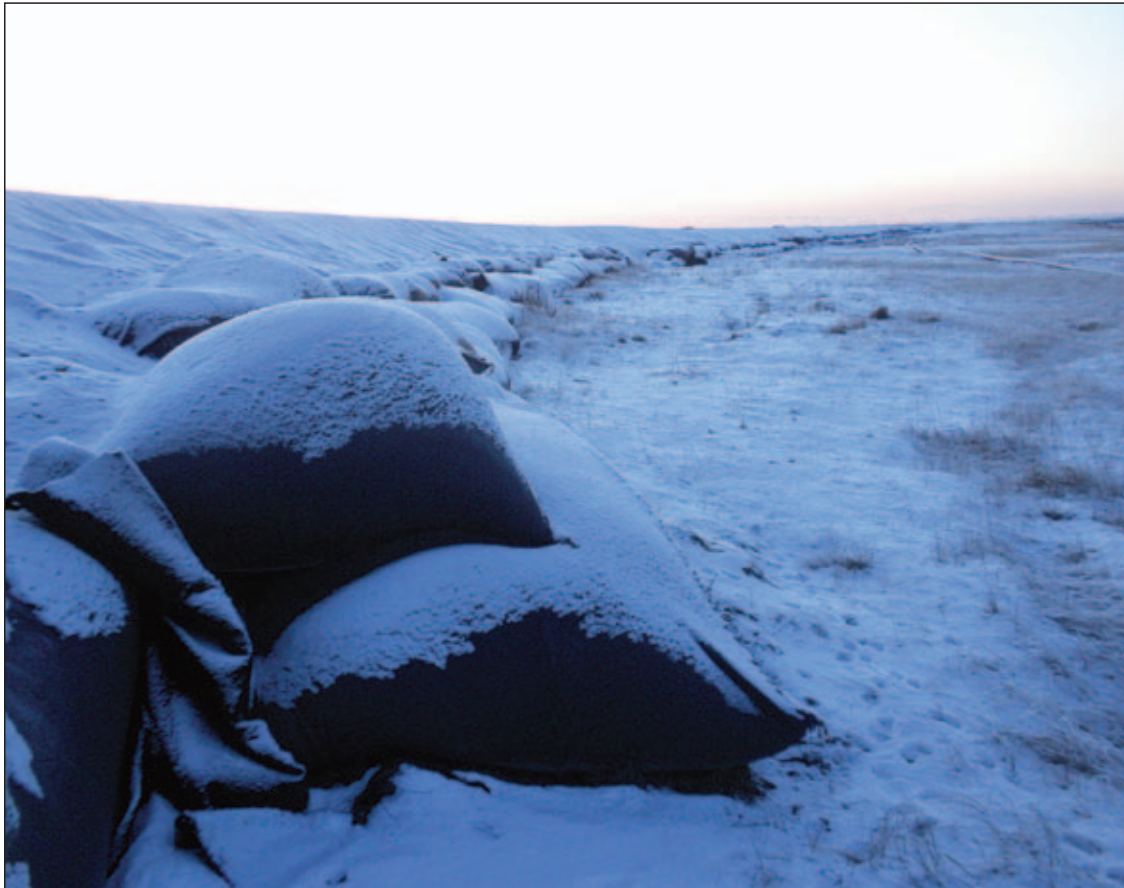
Evacuation road protection against erosion.
