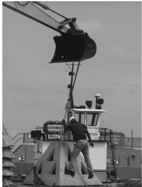
Figure 3. Photograph of coastal havens used at Saw Grass Point Salt Marsh on Dauphin Island, Alabama.
