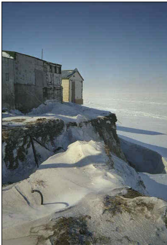
Figure 7. Photo of coastal erosion leaving buildings at the edge of the sea at Shishmaref, Alaska.
