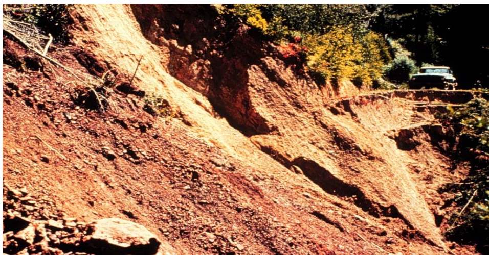
Figure 1. Photo of a roadcut failure. Cut banks on rural roads are often very close to vertical. These banks are more prone to failure as warmer more intense winter storms increase proportion of rain versus snow. Access to rural locations will be lost more frequently and roadway maintenance costs will rise.
