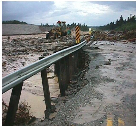
Figure 3. Photo of channel and bridge repairs after a flash flood at One Mile Creek.
