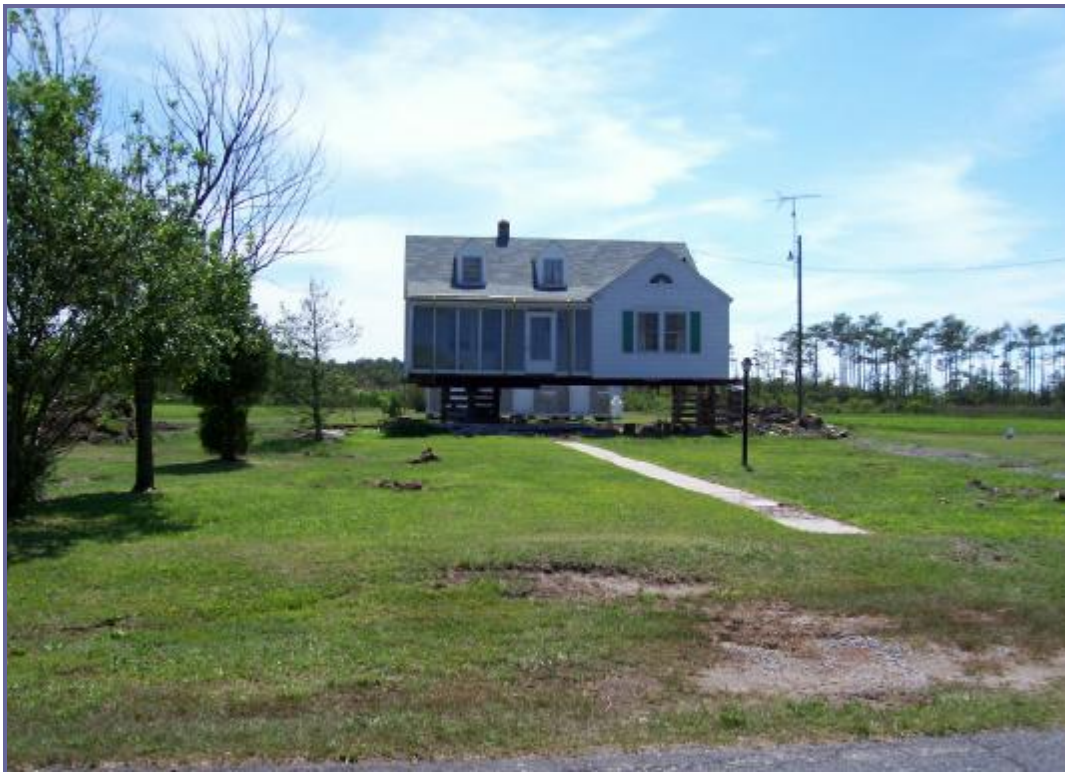
A Toddville Road home damaged by Tropical Storm Isabel in 2003 is elevated using FEMA funds in 2006. From the road, appearances are deceiving; behind and across the street from the house are extensive areas of high marsh and tidal channels. Toddville, Maryland 2006
