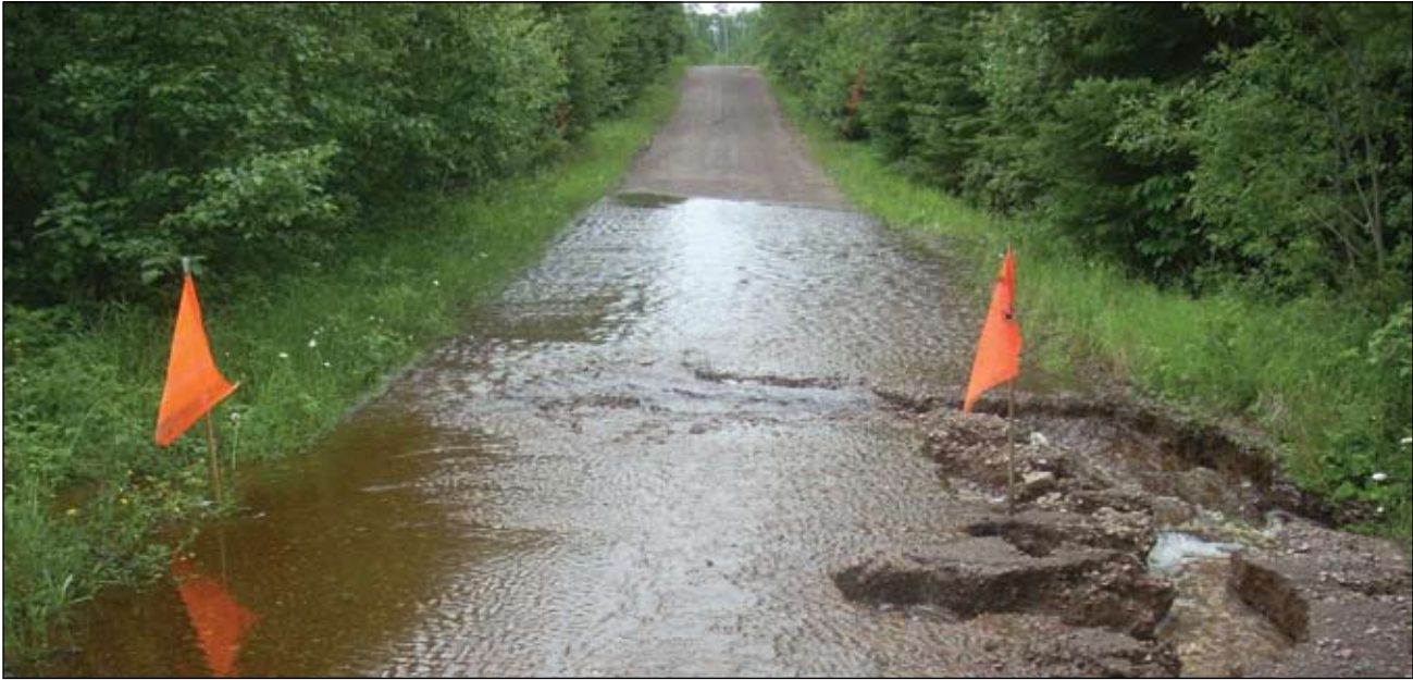
Water running over a forest road following the June 2012 rainstorm in northeastern Minnesota. Photo by Patrick Hampston, Superior National Forest.
