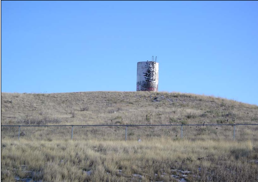
Water storage tank for Busby
