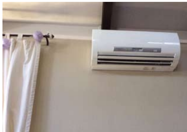
The indoor unit for a ductless heat pump can be installed without significant construction. Photo: Sara Thompson via Flickr CC BY-SA 2.0.
