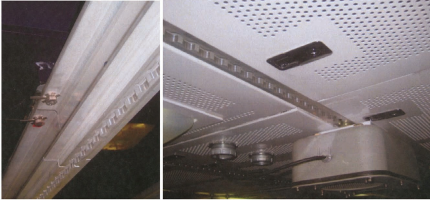
Figure C.3 Flexible Infrastructure Overhead Track System
