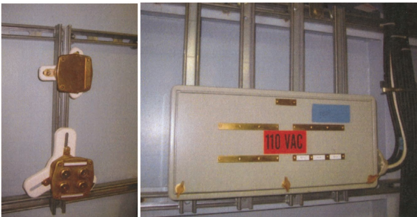
Figure C.2 Flexible Infrastructure Bulkhead Track System
