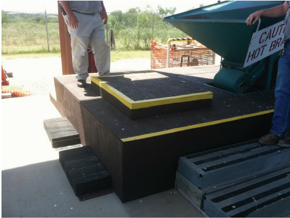
Figure C.2. Steps and Platform Installed for Brass Deformer
