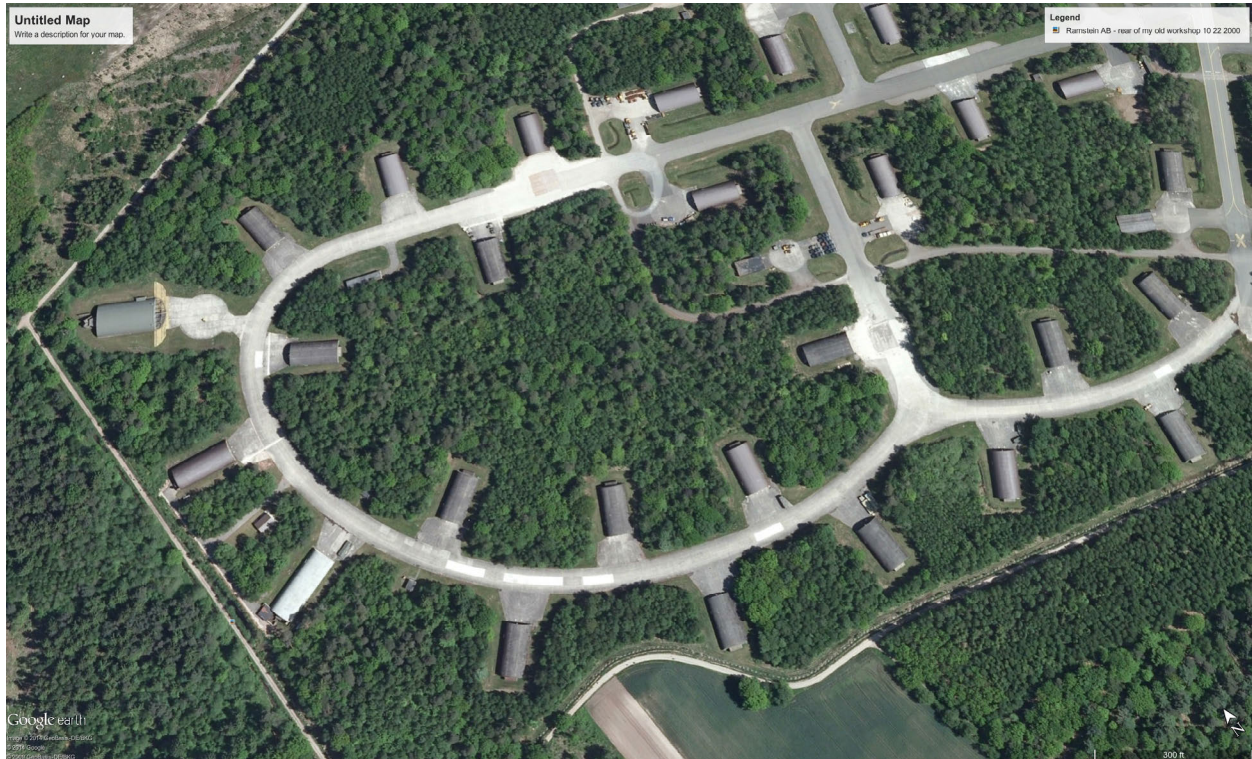
Figure 5.1. Hardened Aircraft Shelters on Loop, Ramstein Air Base, Germany
