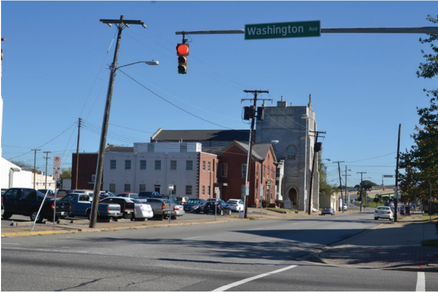
Figure 3.6 A Parking Lot near Newport News Shipbuilding
