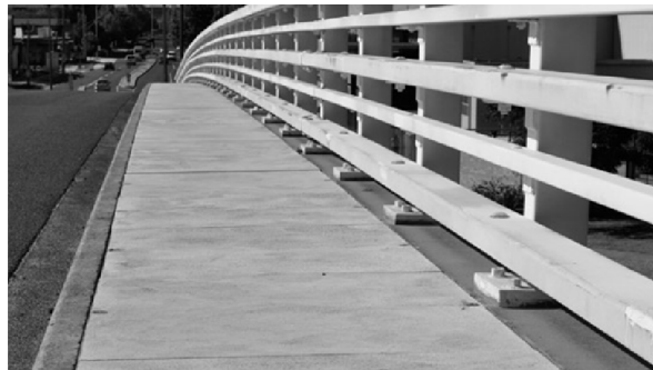
Figure 30: Geopolymer concrete used for paving.
