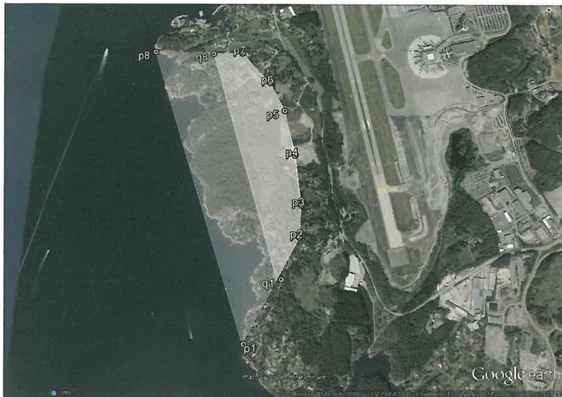
Figure 9: Example of excavation and mass filling close to Bergen Airport Flestrand. Google map.
