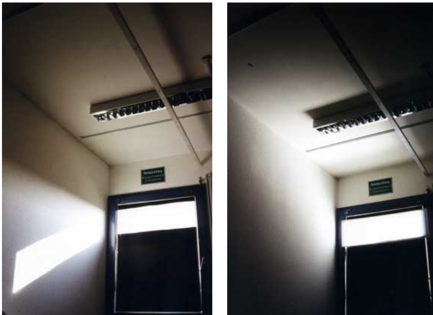
Figure 5-17. Illustration of light distribution in a side-lighted space without (left) and with (right) sun-directing glass in the clerestory portion of the window. Pictures from the web-site of the company LIFLITE GmbH; www.liflite.de
