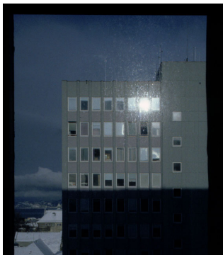
Figure 2-6. Reflected sunlight from a solar shading device causes glare problem in a north-oriented office in the opposite building.
