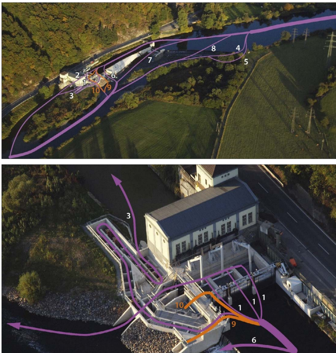
Figure 3.3. The different routes downstream migrating fish can use to pass the Unkelmühle power station: 1) via custom-made openings in the racks that leads fish to a route outside the turbines via the flushing channel, 2) through turbines if they slip through the bar spacing of the racks, 3) through the vertical slot fish passage constructed for upstream migrants, 4) through the nature-like fishway, 5) through the canoe pass, 6) via the ice gate, 7) over the spillway gate, 8) over the dam, 9) via the bottom bypass for eel, and 10) via side bypasses for eel (the two latter, indicated in orange, are only in operation during the eel run in the autumn). Numbers in both panels refer to the different migration routes. Photos: Wikimedia Commons.
