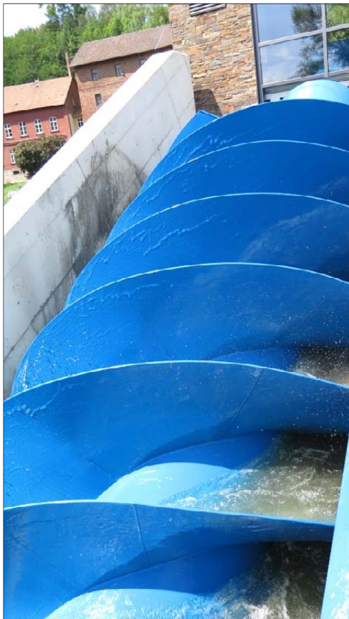
Figure 6.1. The Archimedes screw turbine at Kuhlemühle in the Diemel.
