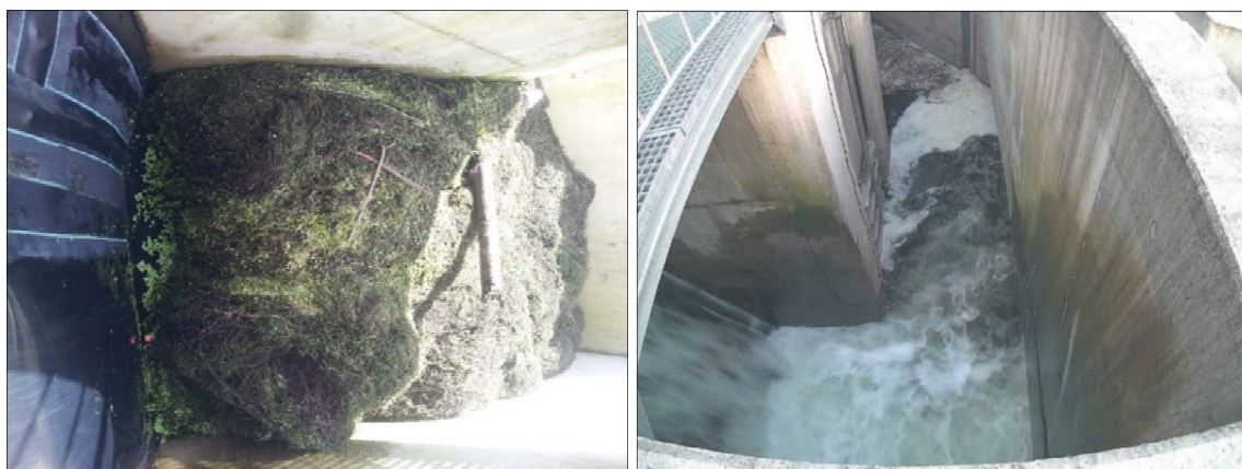
Figure 4.3. Area of the bypass route outside the turbines at the Unkelmühle power station where debris and branches were piling up in 2014 and likely caused mortality in Atlantic salmon smolt that were trapped (left). There was no debris piling up and no recorded mortality at this particular site during the study in 2015 (right). Photo: Finn Økland and automatic monitoring camera.
