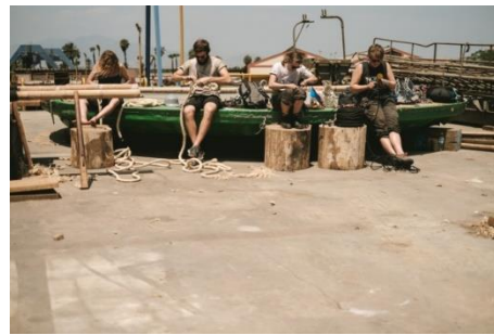
Figure 2 The floor of the deck was made of bamboo logs tied next to each other (left). Skilled knot tiers and a hard-working building team assembled both the deck and the cabin with the same material.
