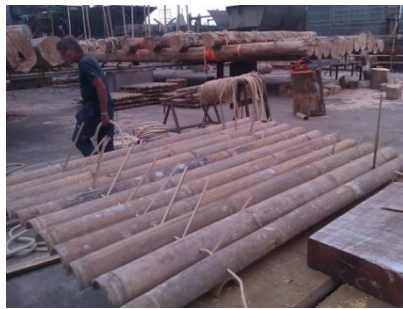
Figure 2 The floor of the deck was made of bamboo logs tied next to each other (left). Skilled knot tiers and a hard-working building team assembled both the deck and the cabin with the same material.
