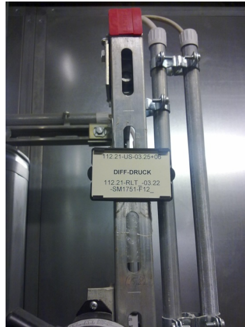
Figure 2.9 Label on Field Device
