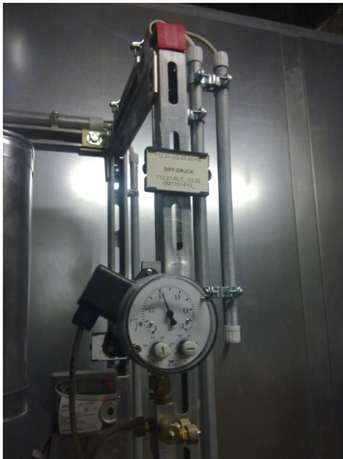
Figure 2.8 Field Device with Data Point Address
