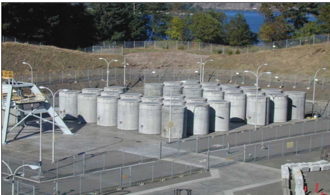
Figure 1 Dry Storage. Source: Portland general electric Co.
