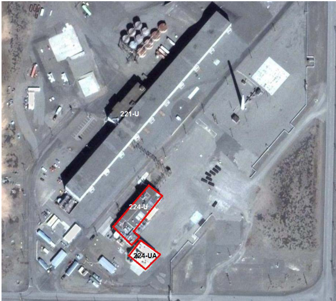
Figure 1.1. Aerial View of the 224-U and 224-UA Buildings and Surroundings Before Demolition
