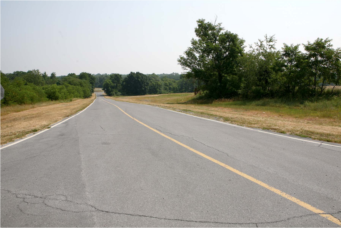
Figure 7. Most of the roads on the Depot have shoulders that are mowed making the placement of gas collection systems in these areas a very viable option.
