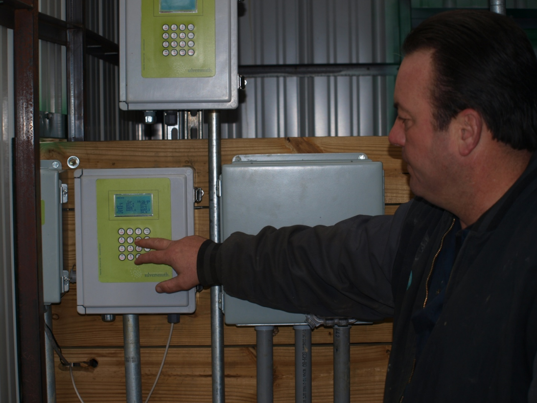
Figure 17. Frank Irvin explains how the gas metering and monitoring system is computer-controlled.
