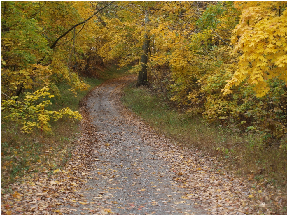
Figure 13. Location of gas collection system buried either under or alongside existing roads.
