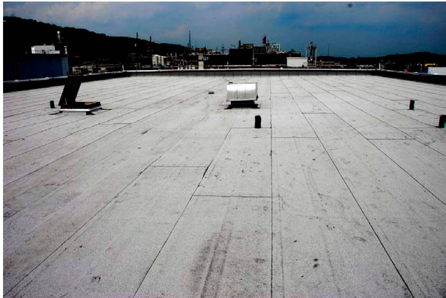
Fig. 1.6. All future roof replacements will use the cool roof technology.
