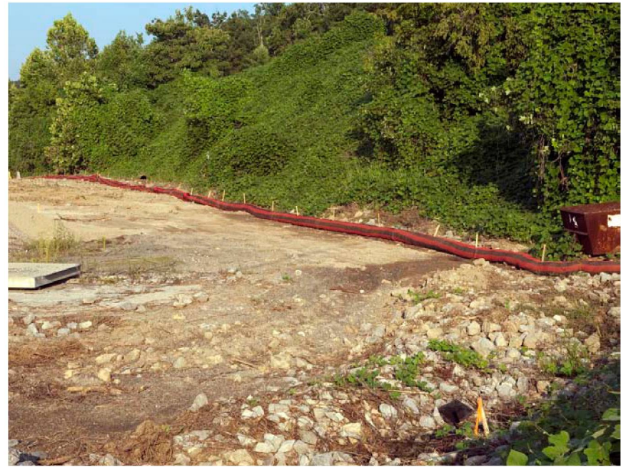
Figs. 5.2 and 5.3. Approximately 1500 yd 3 of mulch was created from trees and brush that were cleared during construction of a new bypass road. This mulch was then put inside fabric bags for use as erosion control devices. This project illustrates the reuse of natural resources in order to protect other natural resources.
