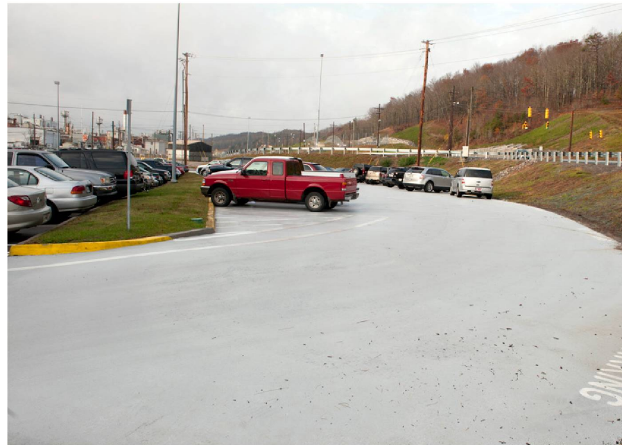
Fig. SIGS.1. The site continues road and grounds planning for new parking lots and road construction using porous pavement, warm-mix asphalt, and rolled compacted concrete as sustainable options
