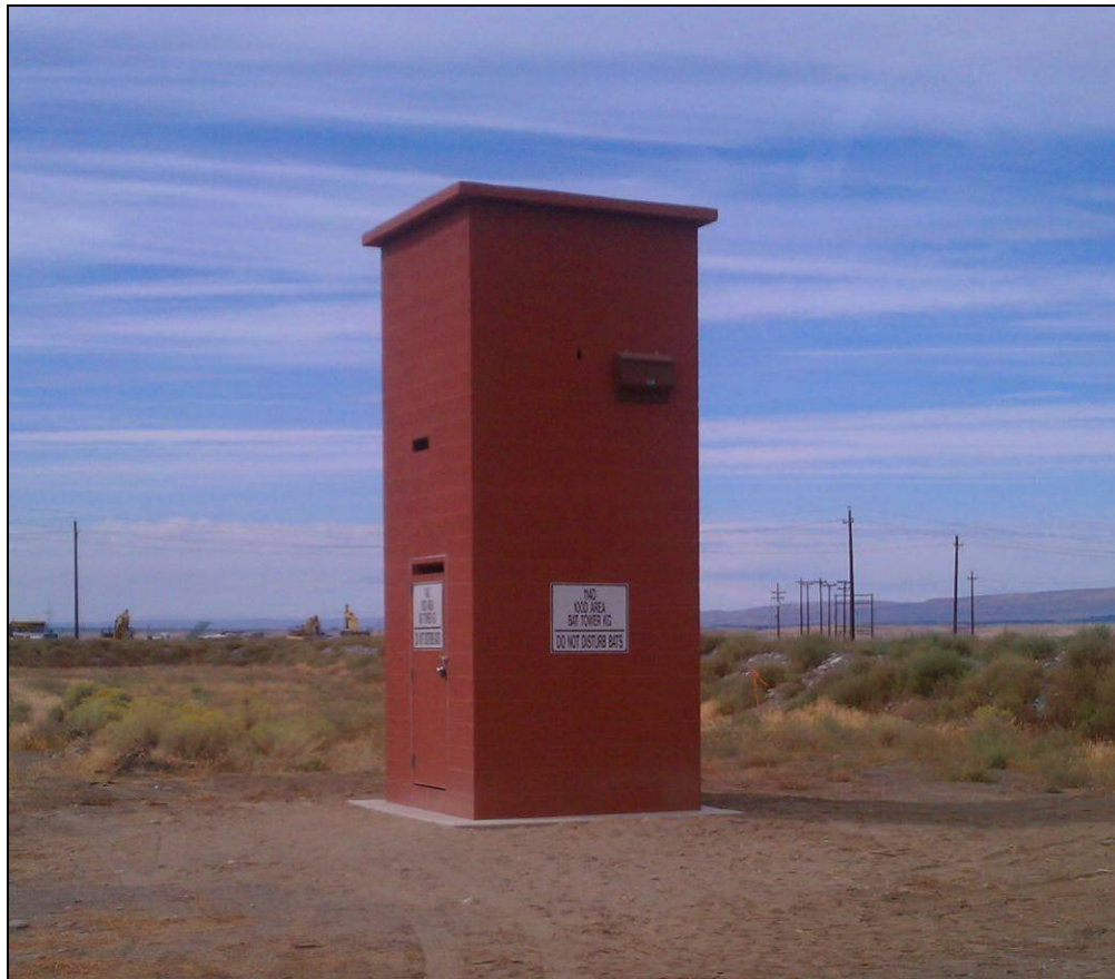
Figure 26. Artificial Bat Roost at 100-D Constructed in 2011.
