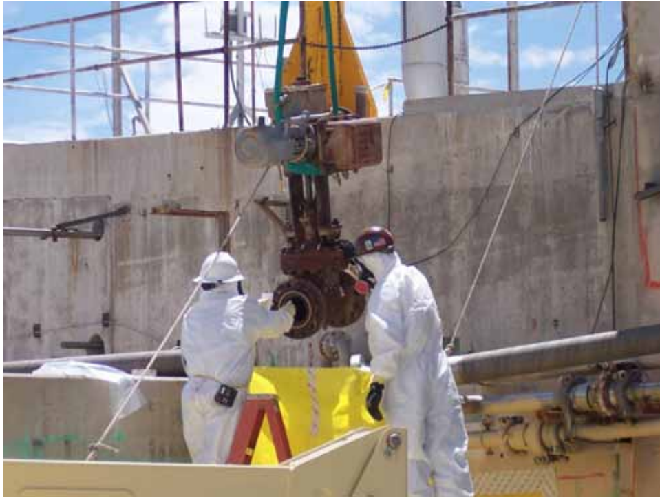
Photograph 13: Removal of Nuclear Furnace Piping, 07/22/2009
