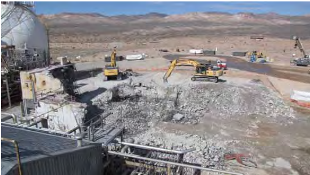
Photograph 40: Demolition of Building 3210, 02/15/2011
