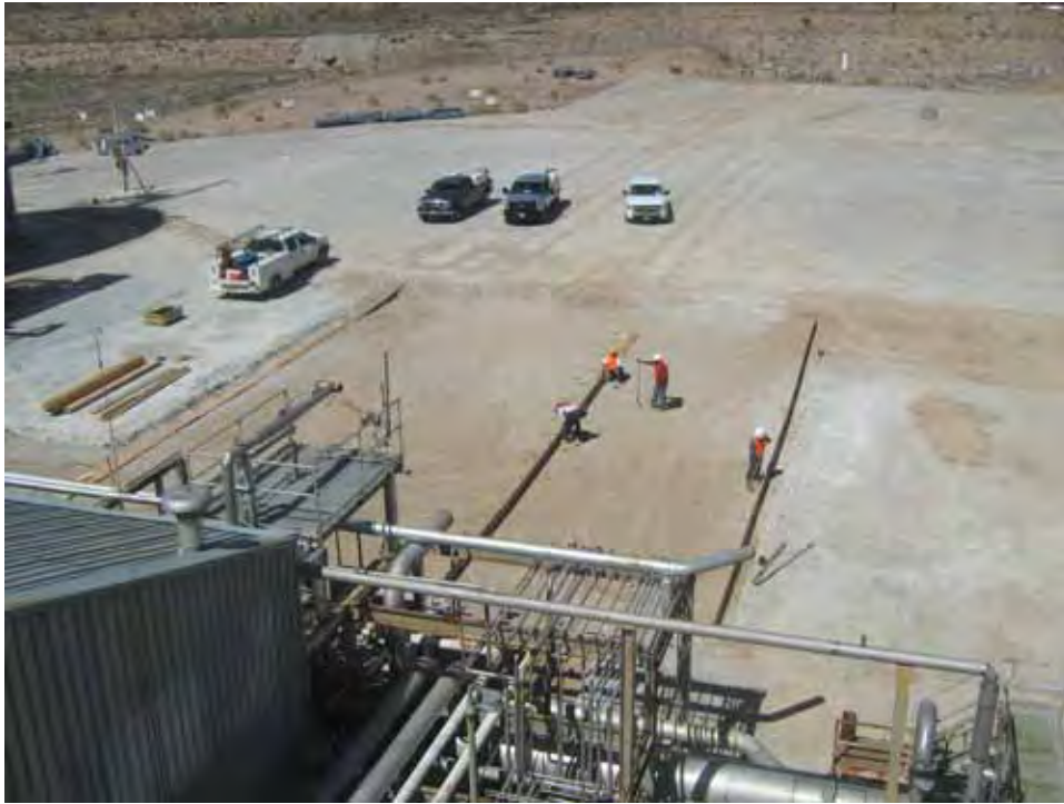
Photograph 45: Preparation of Basement for Placement of Concrete, 03/30/2011
