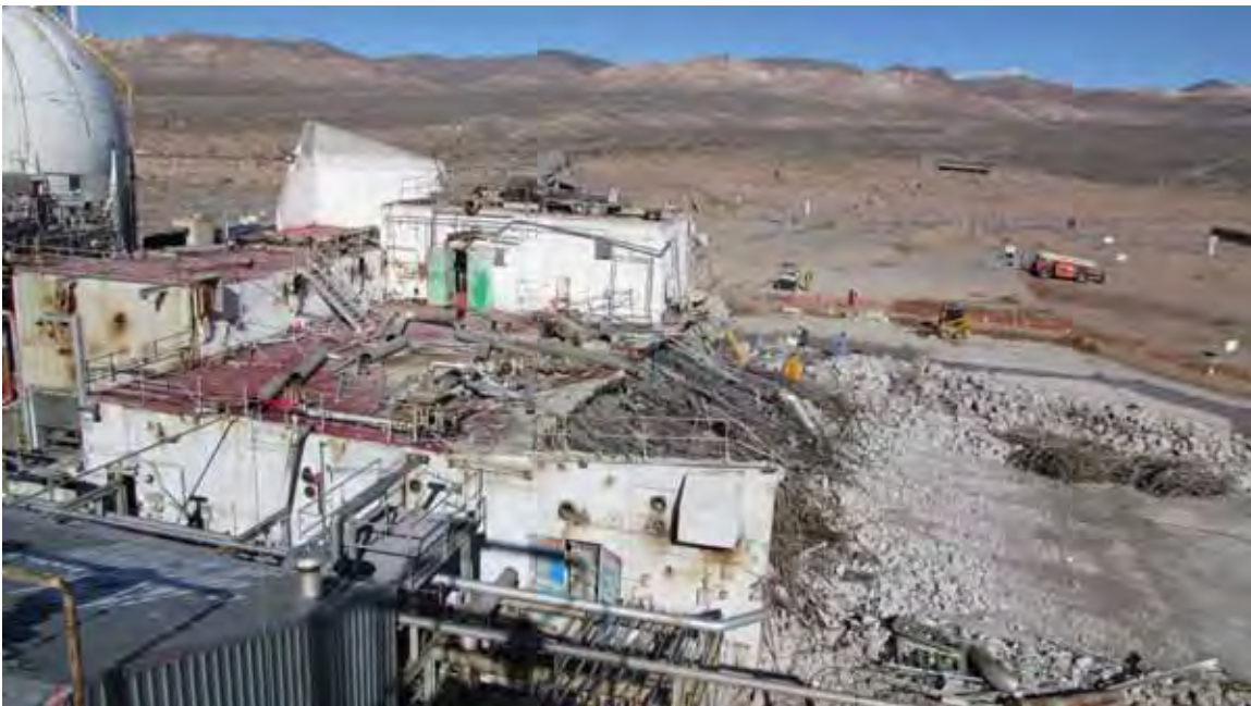
Photograph 32: Demolition of Building 3210, 01/06/2011
