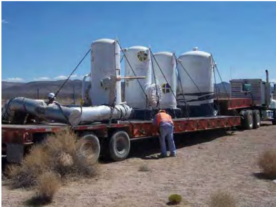
Photograph 16: Tanks Loaded for Disposal, 08/25/2009
