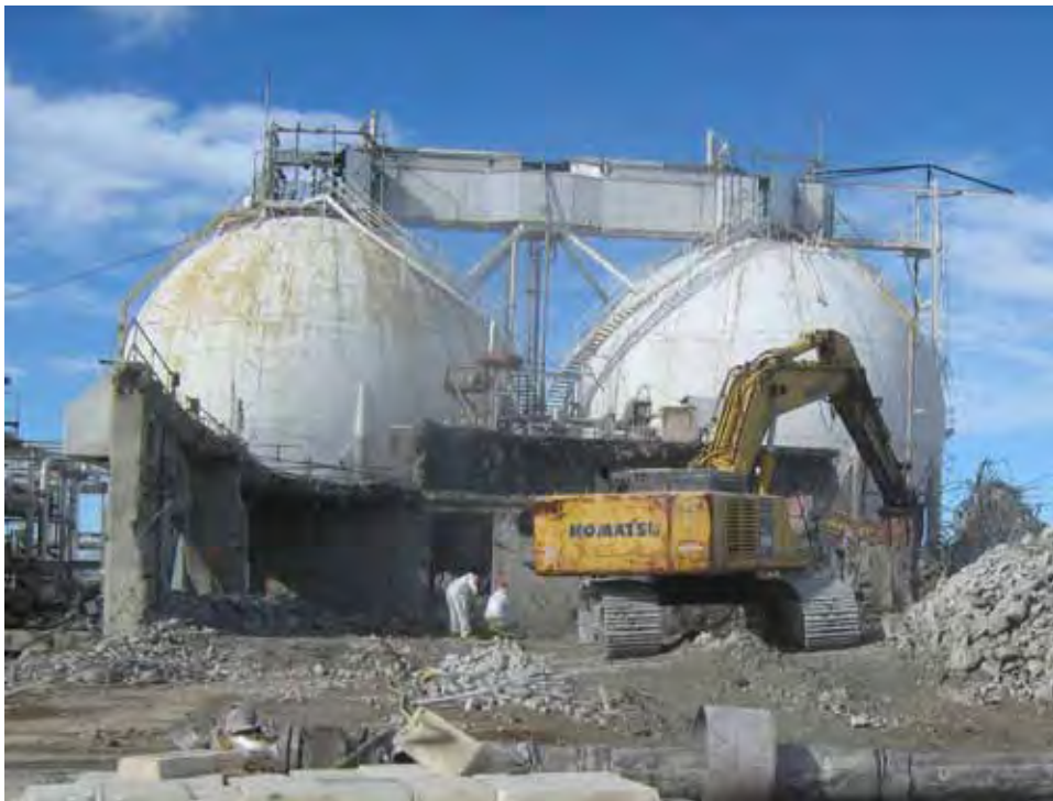
Photograph 38: Demolition of Building 3210, 02/03/2011
