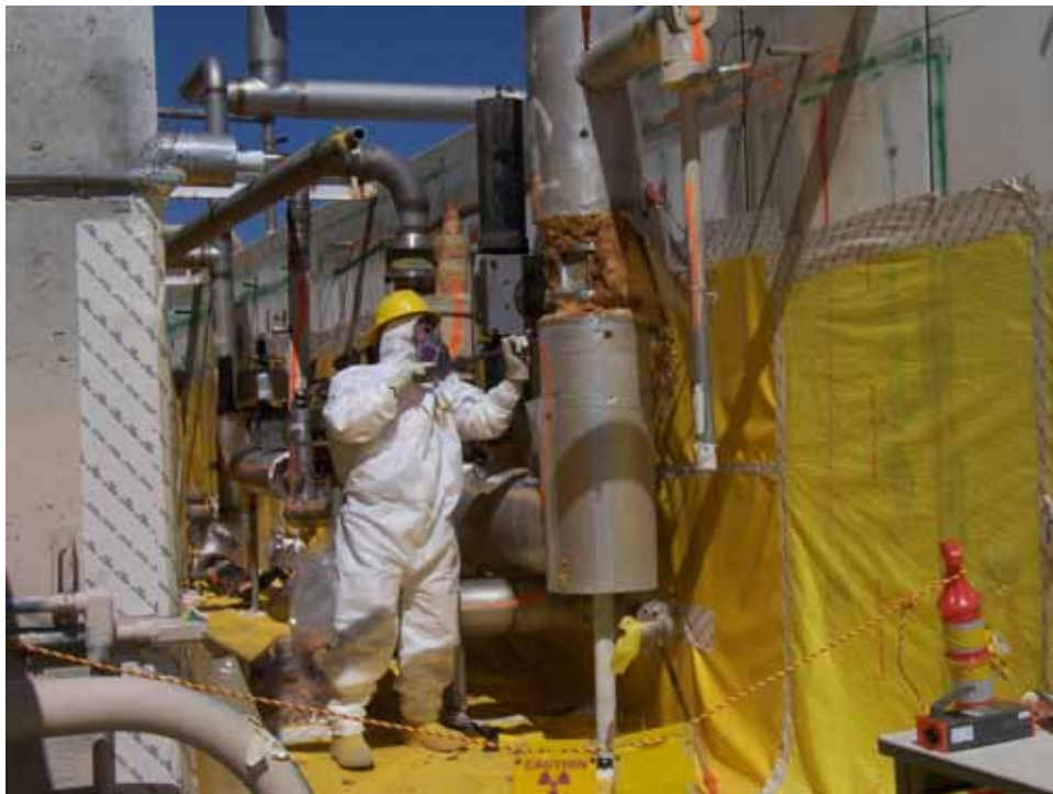
Photograph 14: Removal of Nuclear Furnace Piping, 07/27/2009
