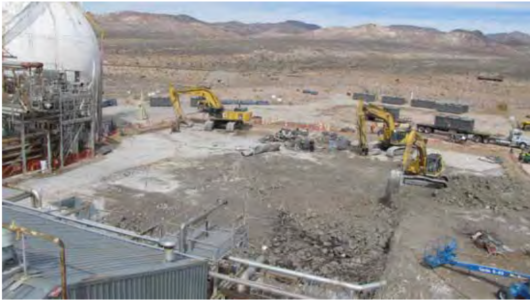
Photograph 43: Demolition of Building 3210, 03/01/2011
