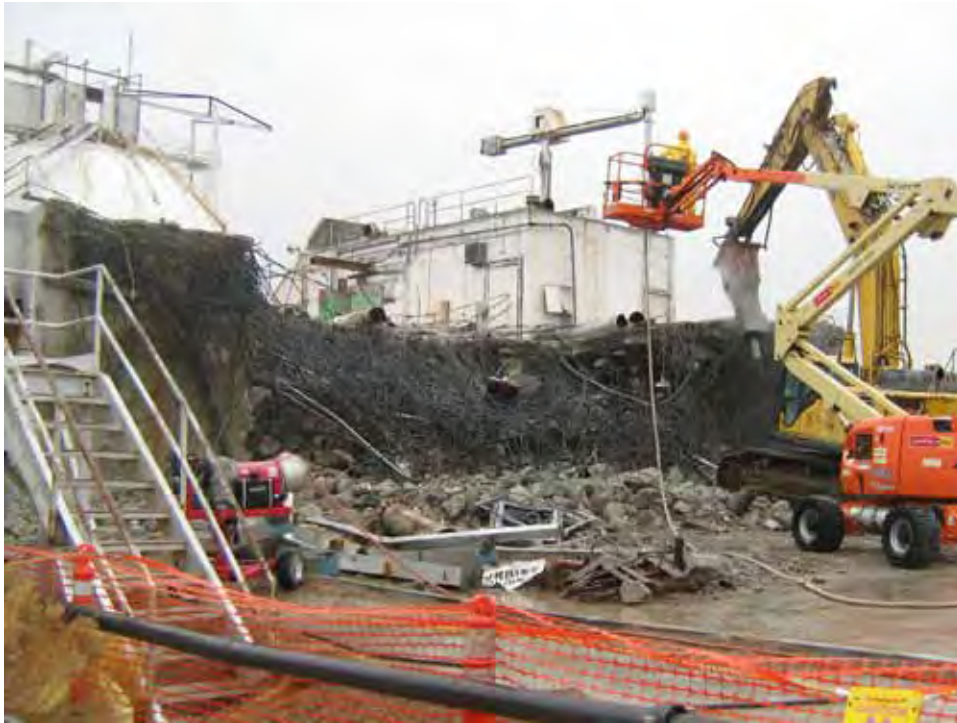
Photograph 29: Demolition of Building 3210, 12/20/2010
