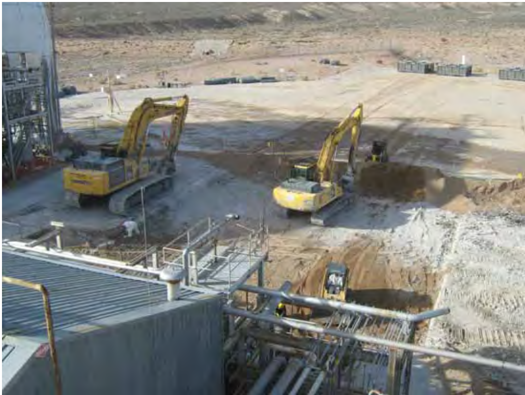
Photograph 44: Backfilling Basement, 03/07/2011
