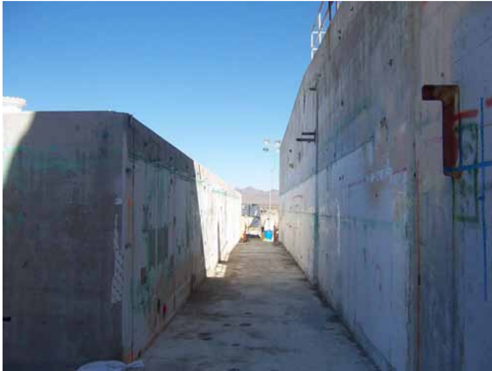
Photograph 17: After Removal of Nuclear Furnace Piping, 08/27/2009
