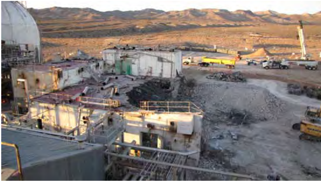
Photograph 35: Demolition of Building 3210, 01/18/2011
