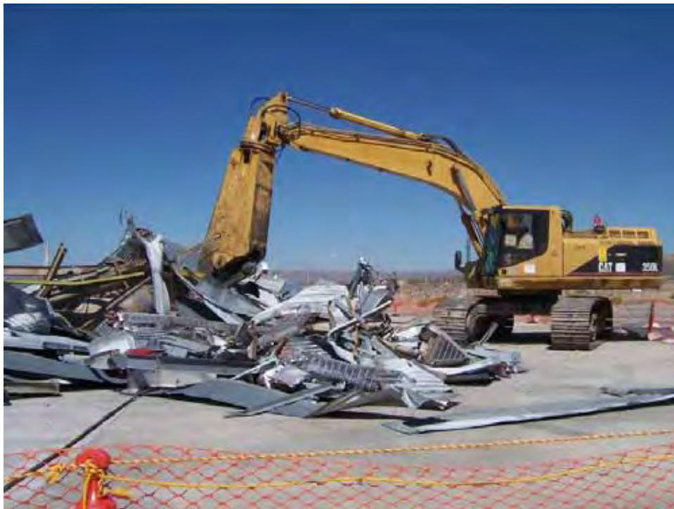
Photograph 10: Size Reduction of Building 3211 Debris, 07/07/2009
