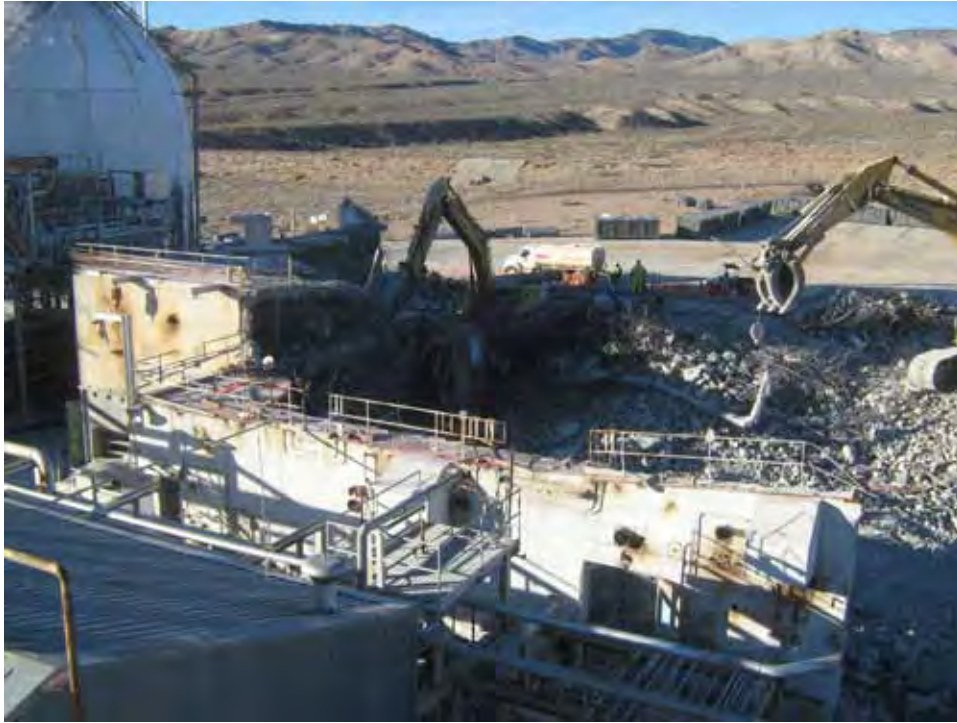
Photograph 37: Demolition of Building 3210, 01/26/2011
