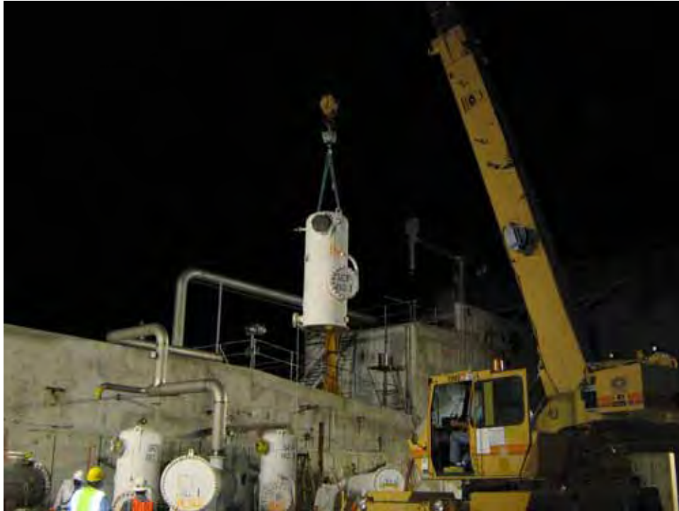
Photograph 15: Removal of Tanks, 08/20/2009
