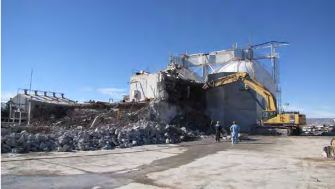
Photograph 31: Demolition of Building 3210, 01/06/2011
