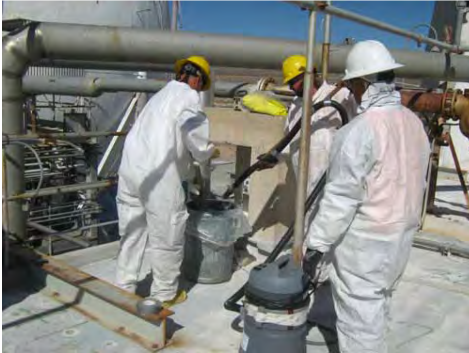
Photograph 21: Removal of Paint Chips from the Roof, 10/14/2010
