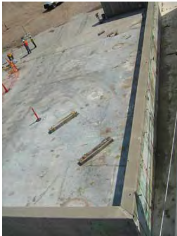
Photograph 18: After Removal of Tanks Associated with Nuclear Furnace Piping, 09/13/2009
