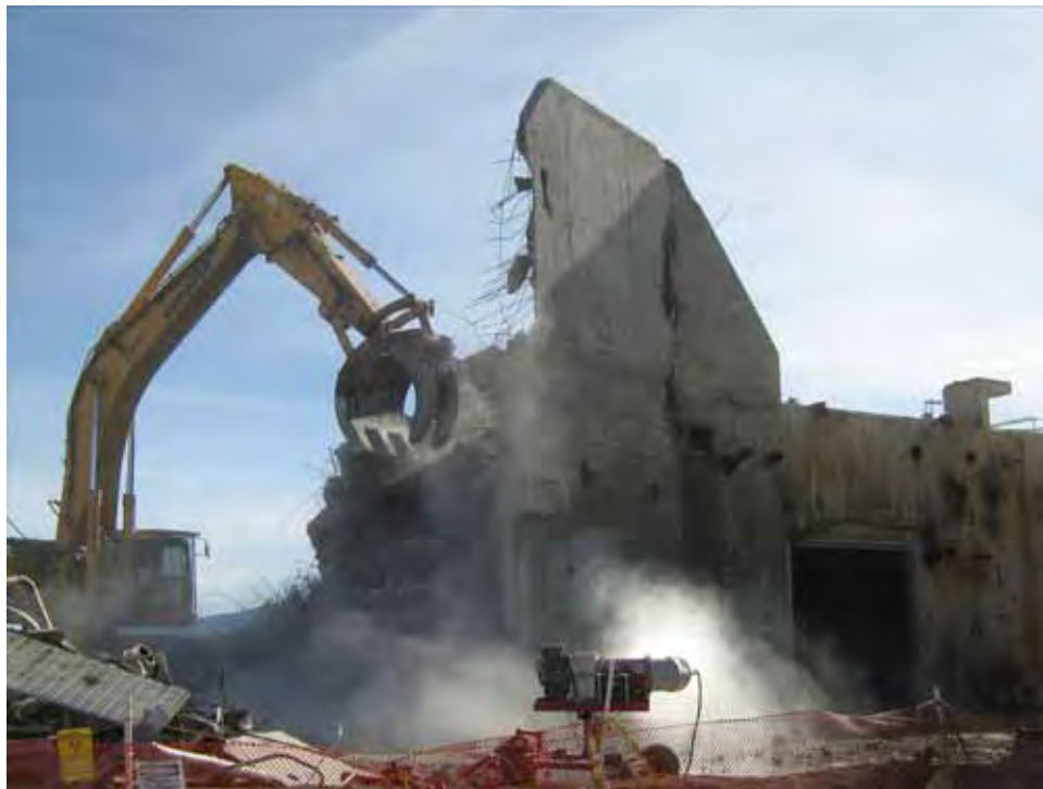
Photograph 34: Demolition of Building 3210, 01/12/2011
