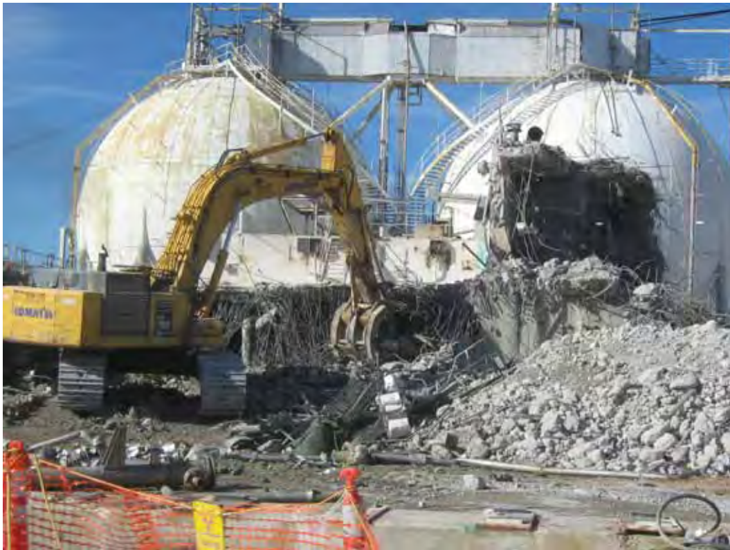
Photograph 36: Demolition of Building 3210, 01/24/2011
