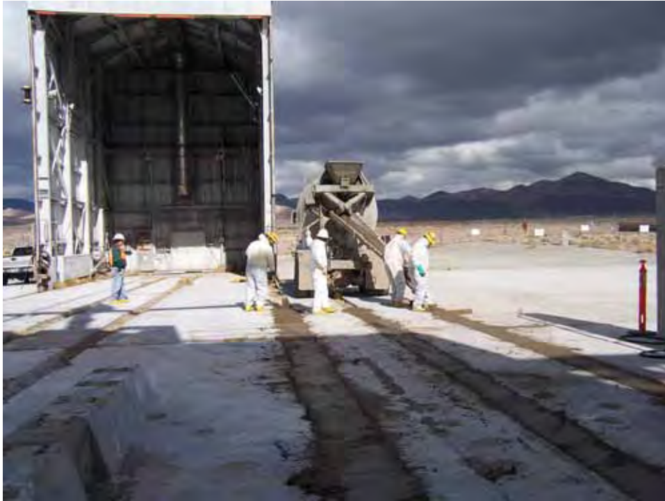
Photograph 3: Grouting Rail Trenches, 01/22/2008
