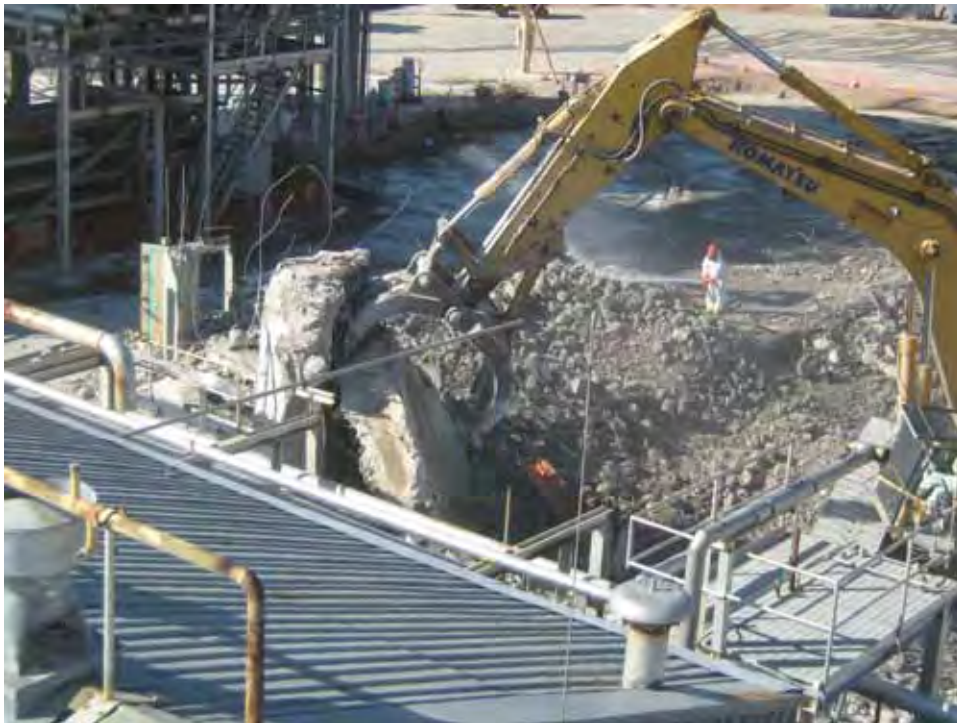
Photograph 42: Demolition of Building 3210, 02/24/2011
