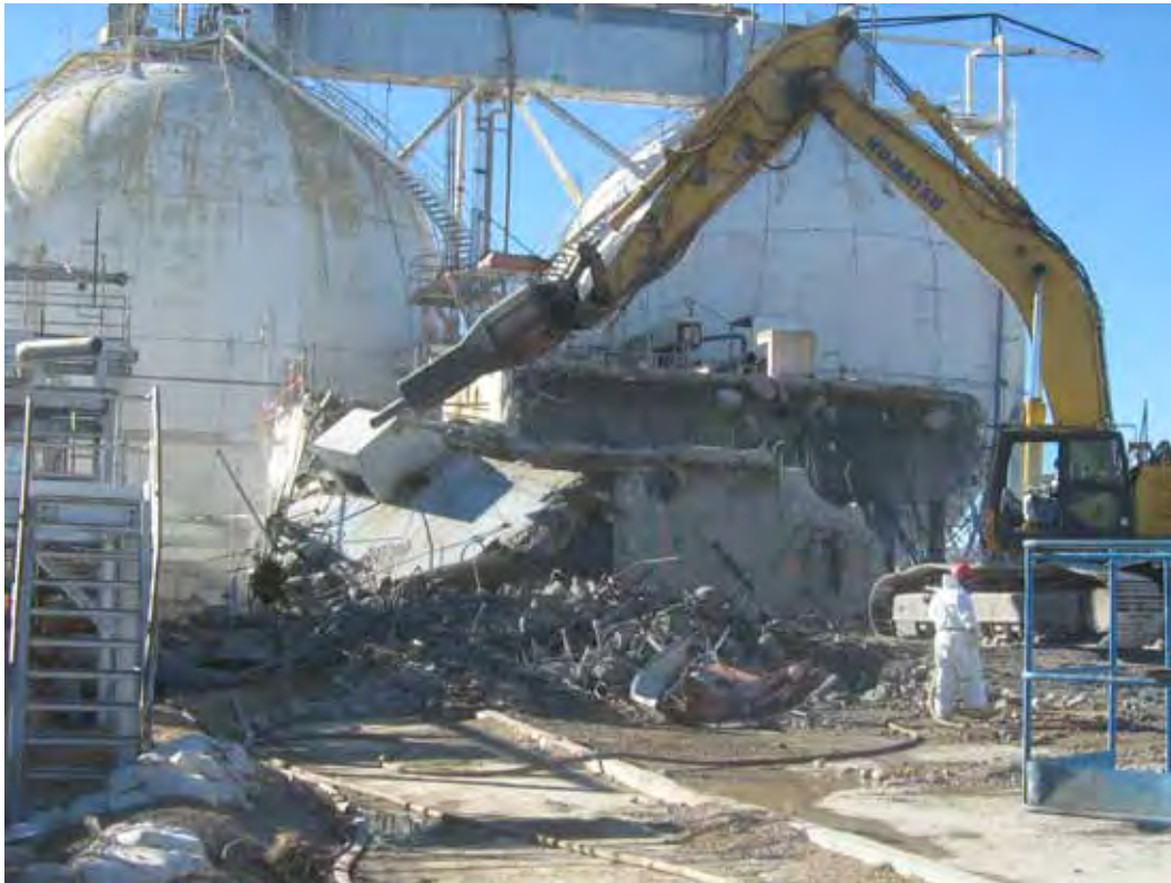
Photograph 39: Demolition of Building 3210, 02/09/2011
