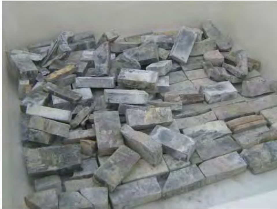
Photograph 33: Lead Bricks Removed During Demolition of Building 3210, 01/11/2011
