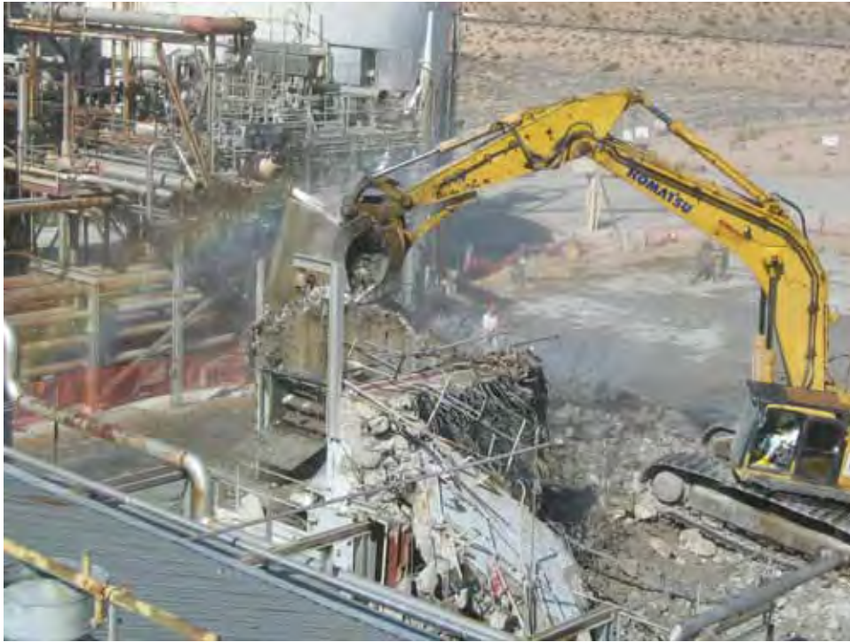
Photograph 41: Demolition of Building 3210, 02/24/2011
