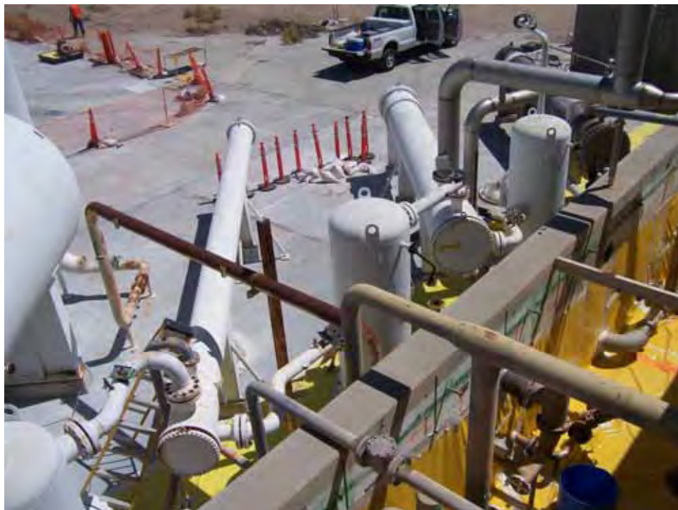
Photograph 12: Tanks Associated with Nuclear Furnace Piping before Removal, 07/21/2009
