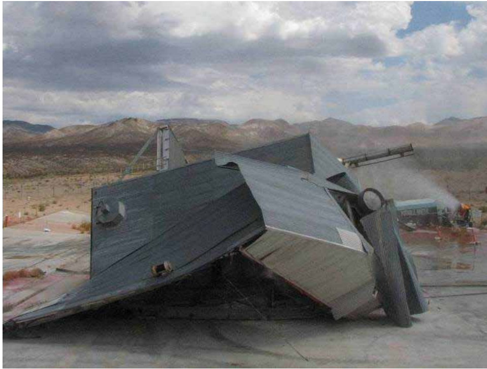
Photograph 9: Demolition of Building 3211, 07/01/2009
