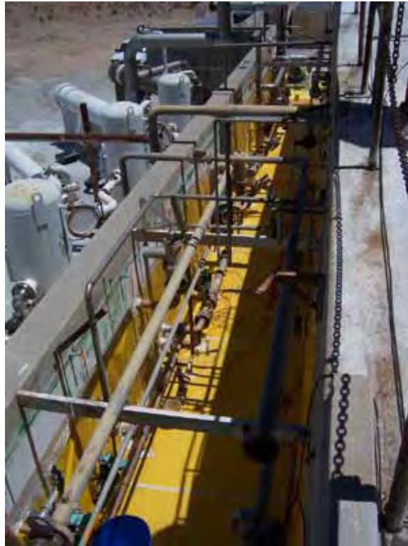
Photograph 11: Nuclear Furnace Piping Area Prepared for Removal, 07/15/2009
