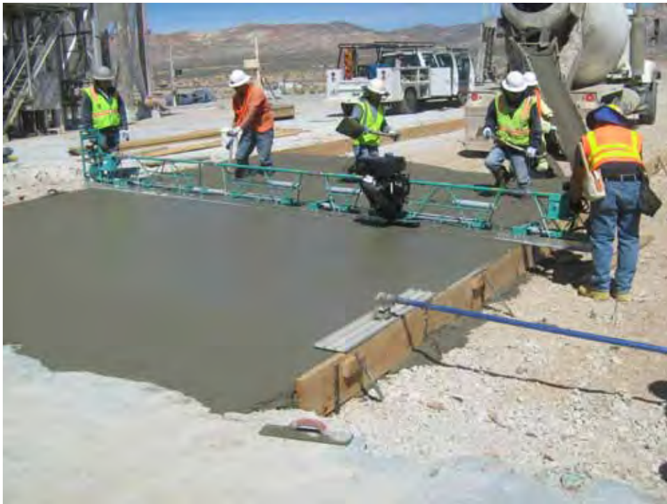
Photograph 46: Placement of Concrete, 04/04/2011
