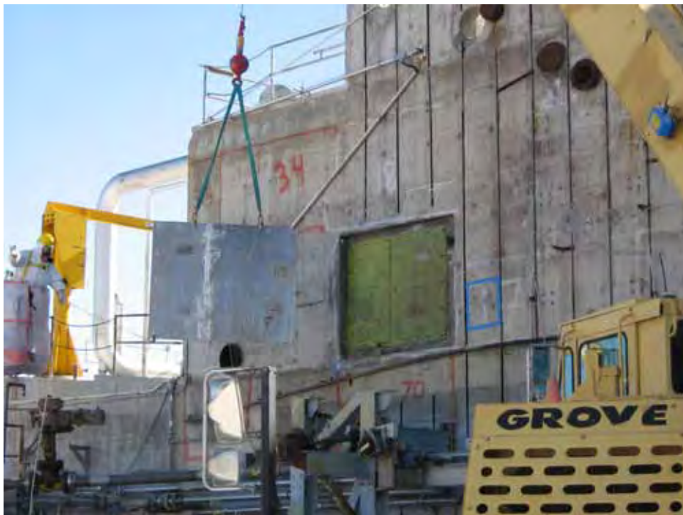
Photograph 4: Lead Sheet Removal, 01/31/2008
