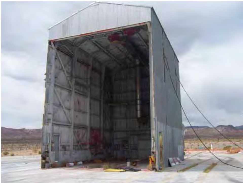
Photograph 8: Building 3211 before Demolition, 07/01/2009
