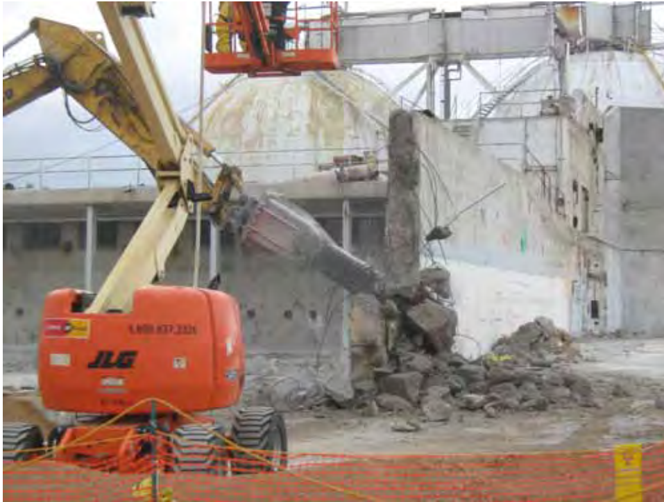
Photograph 27: Demolition of Building 3210, 12/15/2010
