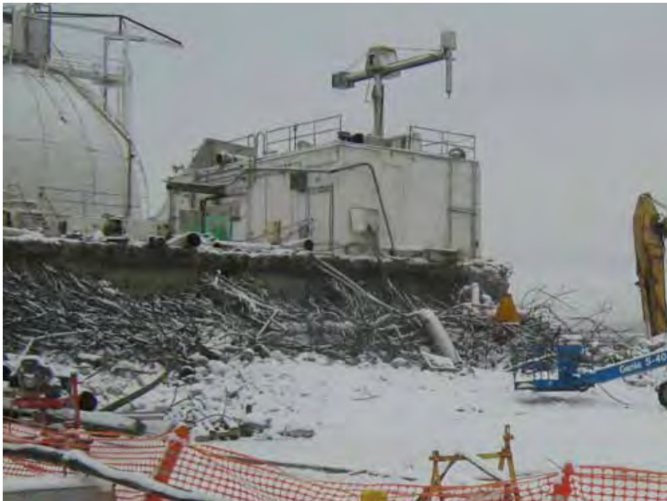
Photograph 30: Demolition of Building 3210, 01/03/2011
