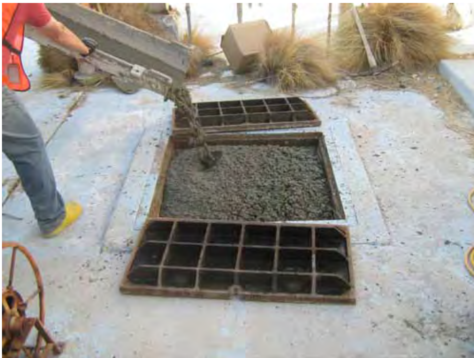
Photograph 22: Grouting Penetrations in the Concrete Pad, 10/19/2010
