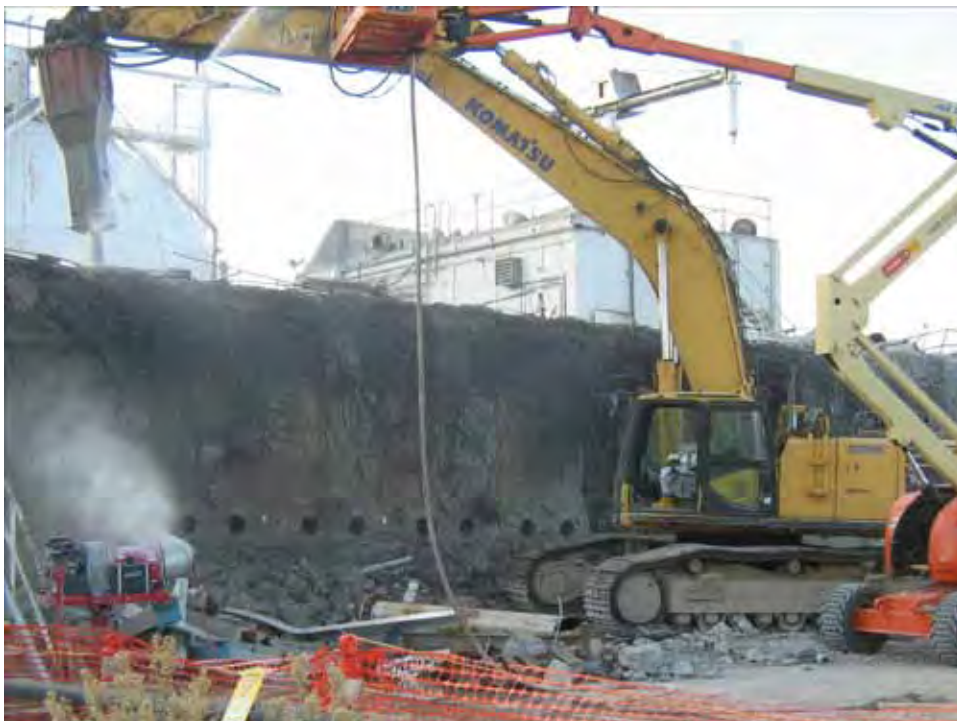
Photograph 28: Demolition of Building 3210, 12/16/2010
