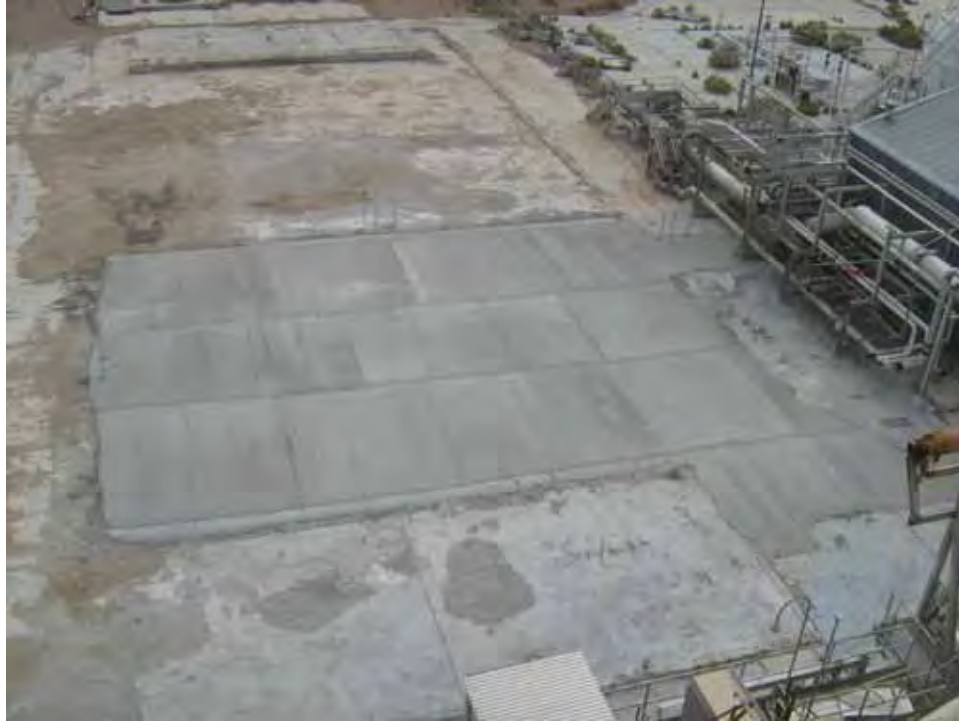
Photograph 47: Grouted Basement, 04/12/2011
