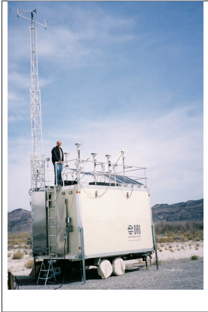
Figure 3. Instrumented mobile shelter at Ash Meadows NWR, showing the meteorological tower with instruments, aerosol sampling inlets, and solar panels.
