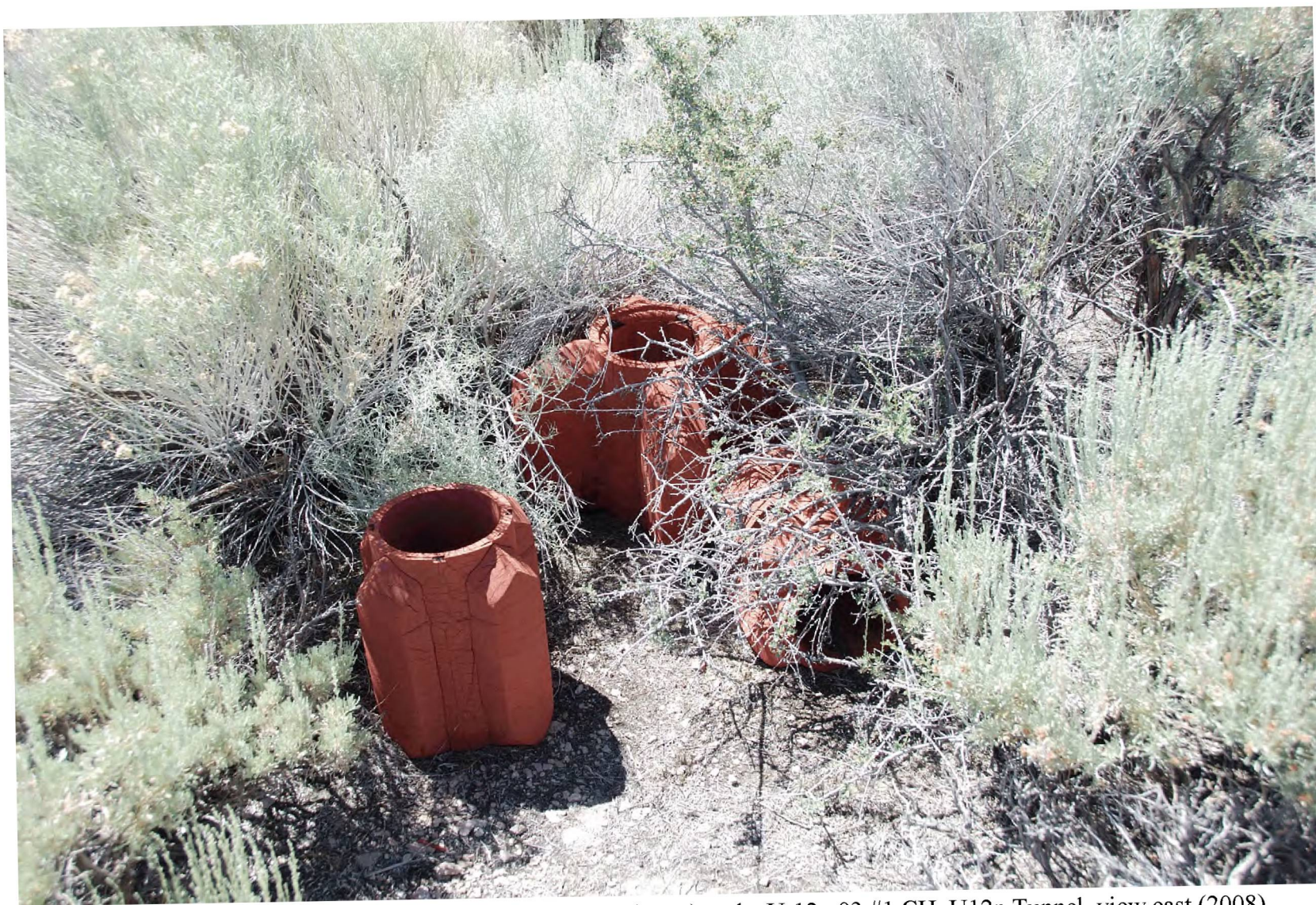
Figure 359. Feature 188, casing centering sleeves (insulators) at the U-12n.03 #1 CH, U12n Tunnel, view east (2008).
