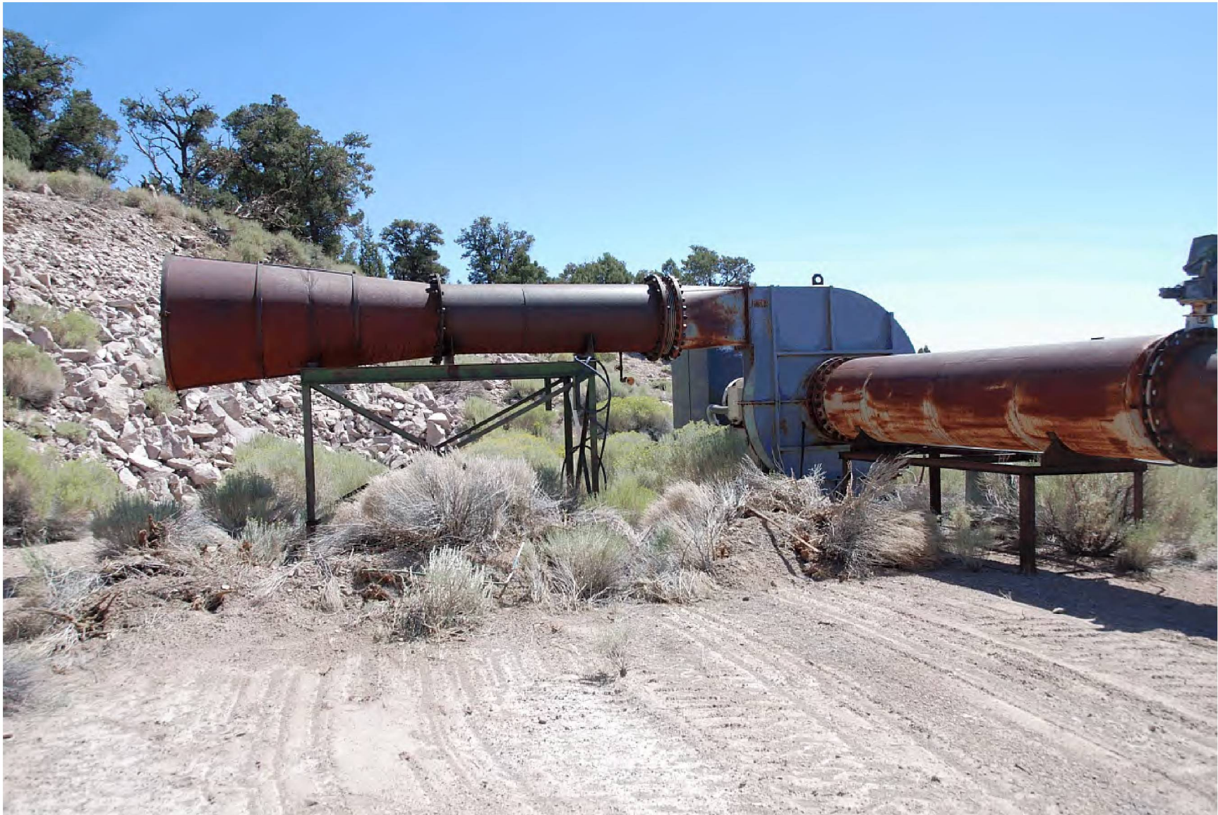
Figure 367. Feature 192, Buffalo Blower and vent lines at the U-12n.10 Vent Hole, U12n Tunnel, view east (2008).
