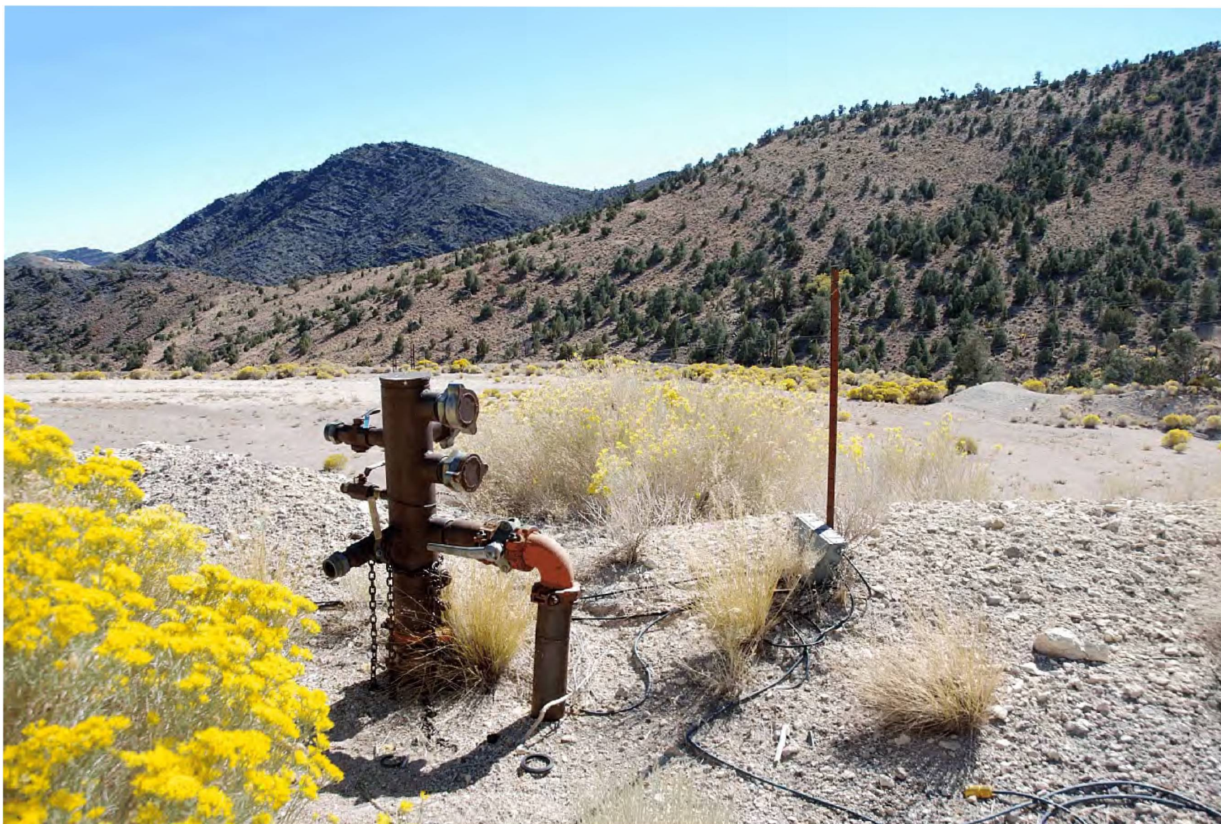
Figure 158. Feature 24, pipe manifold and junction box, U12n Tunnel, view southeast (2008).
