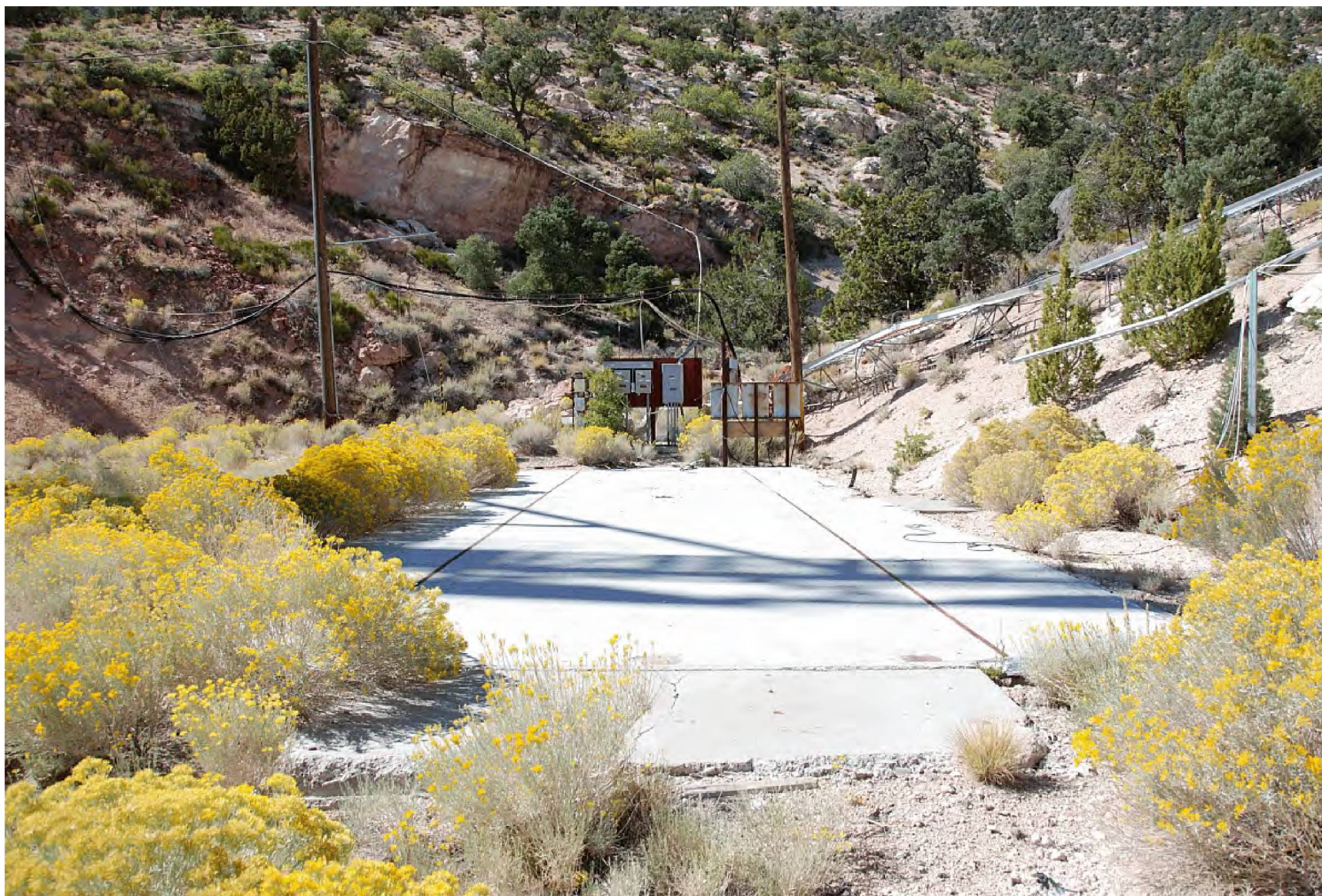
Figure 144. Feature 10, concrete foundation for portal recording station and electrical panels, U12n Tunnel, view west (2008).
