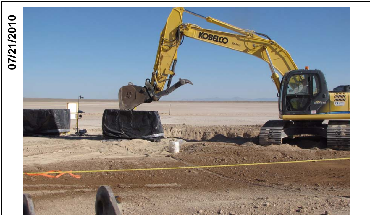
Figure 6-1 Waste Packaging Operations at CA-1 Site
