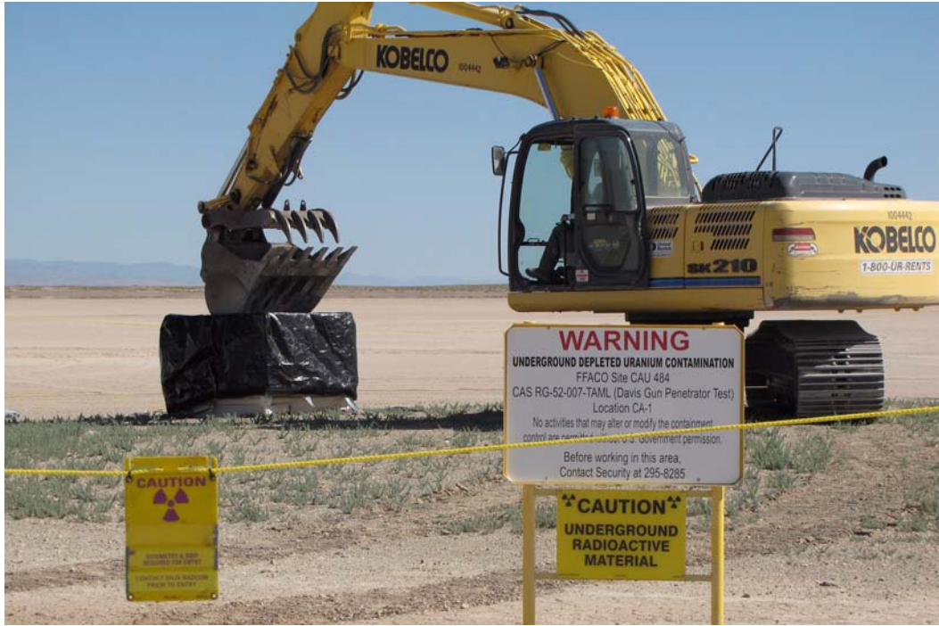
Figure 3-1 Site Setup of Heavy Equipment and Waste Container at CA-1 Site
