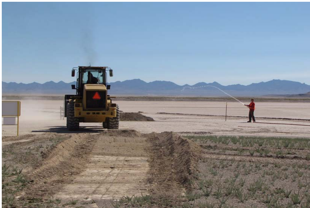
Figure 3-2 Removal of Soil Cap at CA-1 Site
