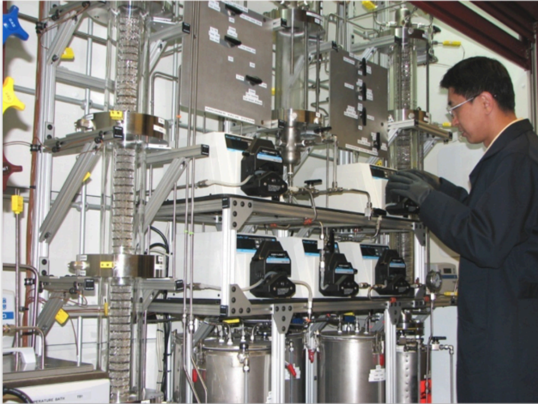
Figure 99: Picture of the installed RSAT simulator used at B&W.
