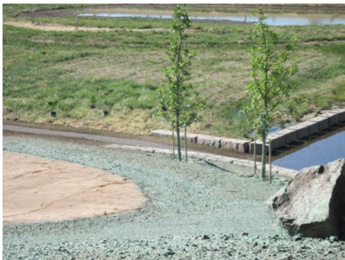
Erosion control blanket and hydromulch stormwater BMPs at the STM campus. Photo by Kurt Schlomberg, NREL/PIX 21210
