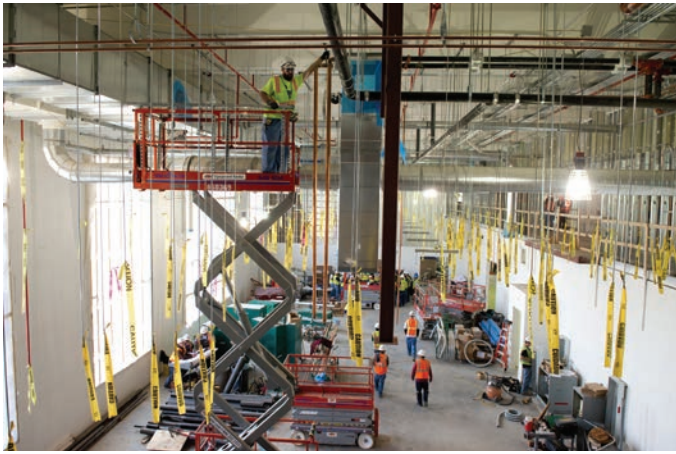
The ESIF laboratory under construction. Photo by Dennis Schroeder, NREL/PIX 20047
