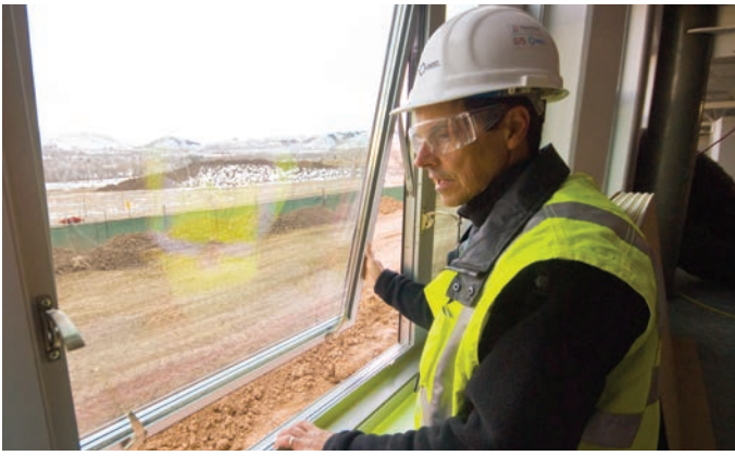
Operable windows minimize use of air conditioning. Photo by Patrick Corkery, NREL/PIX 17092
