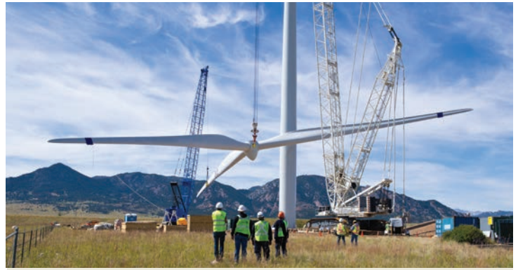
The Gamesa G9X-2.0 turbine assembled at the NWTC is the latest addition to NREL's collection of multi-megawatt wind turbines. Photo by Dennis Schroeder, NREL/PIX 20864
