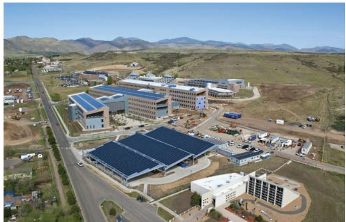
NREL's STM campus. Photo by Dennis Schroeder, NREL/PIX 19095
