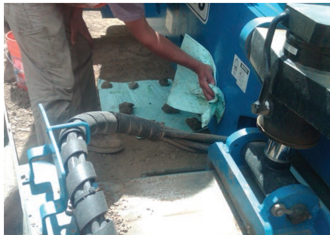
Thorough cleanup of a small hydraulic fluid leak from a boom lift. Photo by Matt Ogle, NREL/PIX 21215
