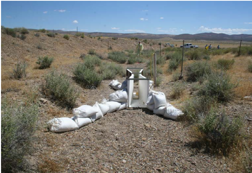
Figure 4. View looking downstream through the flume installed to measure runoff from the Smoky CA.
