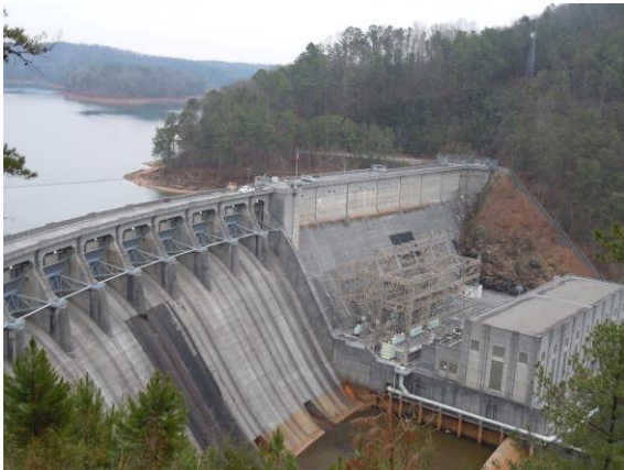
Figure 6: Allatoona Dam and Reservoir, located in northern Georgia, operated by USACE.
