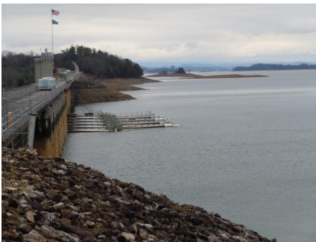
Figure 7: Cherokee Dam and reservoir located in Eastern Tennessee, operated by TVA.
