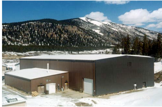
Figure 7. SVP system in Leadville, Colorado
