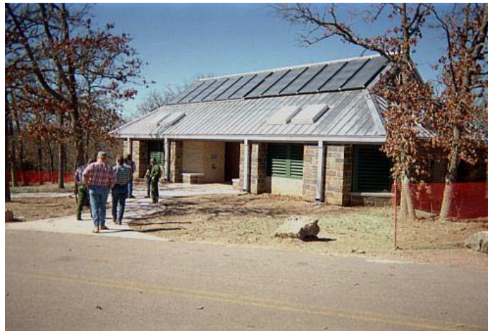
Figure 10. Solar water heating system at Chickasaw National Recreation Area, Oklahoma
