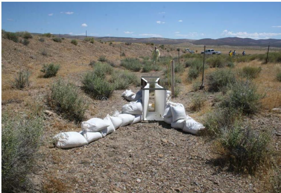
Figure 4. View looking downstream through the flume installed to measure runoff from the Smoky CA.
