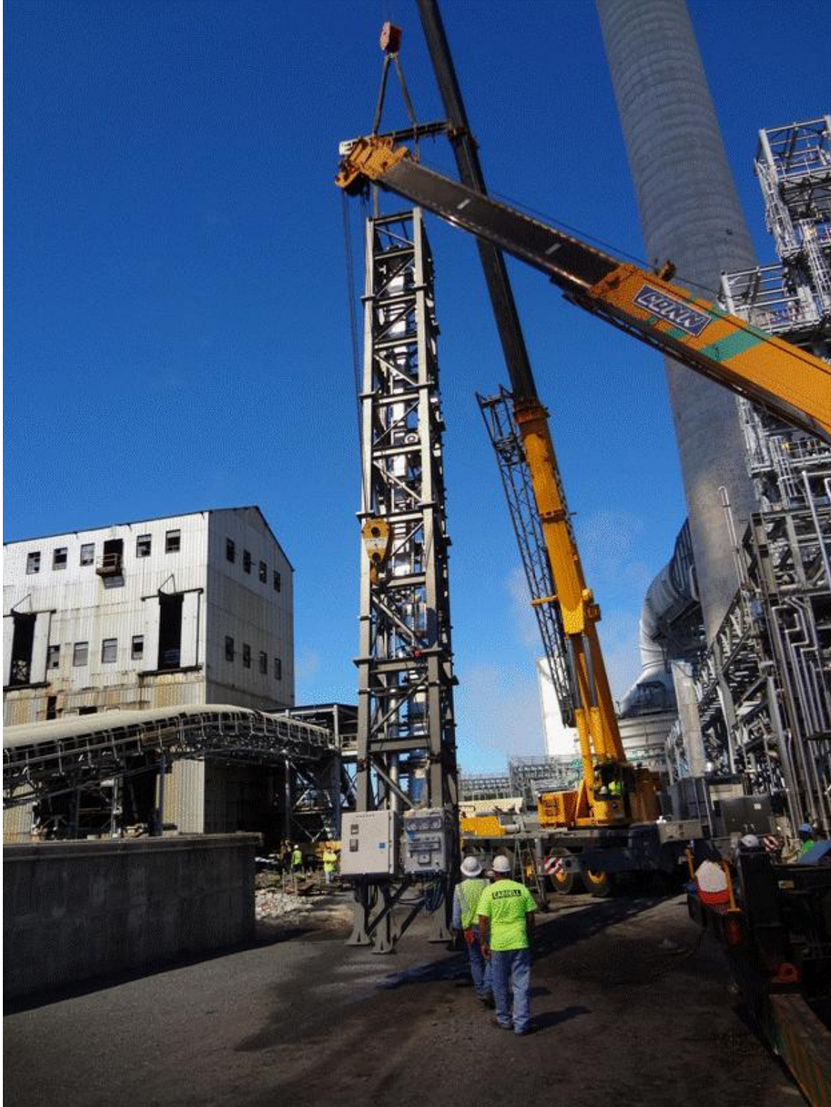
Figure VI-25. The skid lifted from the truck at the NCCC installation.
