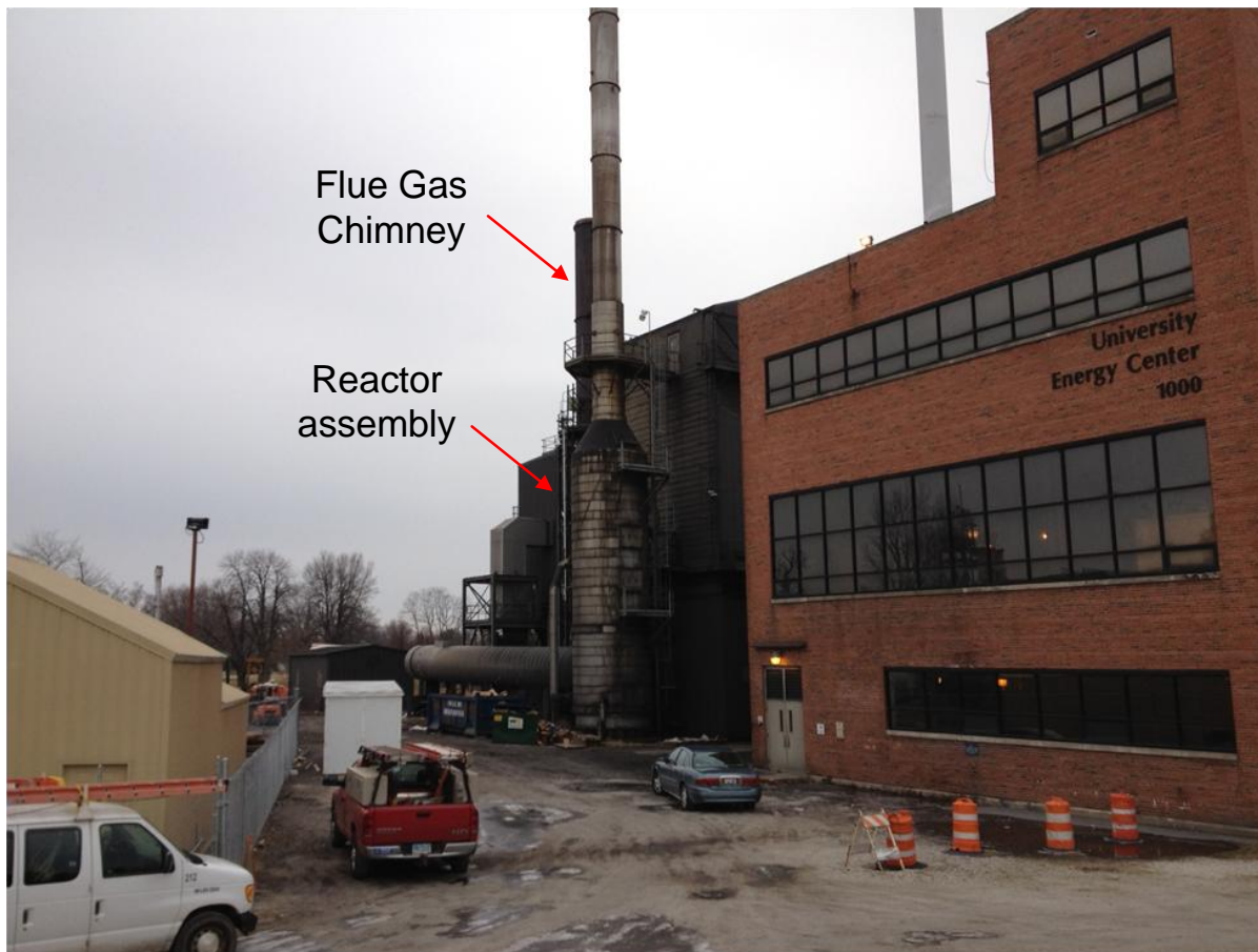
Figure VI-1. The integrated reactor installed at the University of Toledo boiler site.
