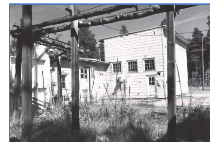
Trinity Test assembly building at V-Site
