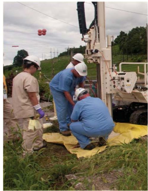
Figure 2-8 Mercury Characterization using Membrane Interface Probe system (Note reduction in the necessary protective clothing)
