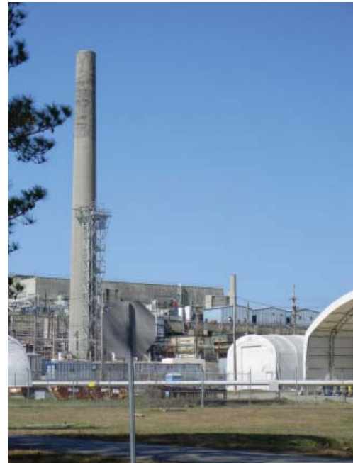
Figure 4-2 Typical SRS Facility Stack
