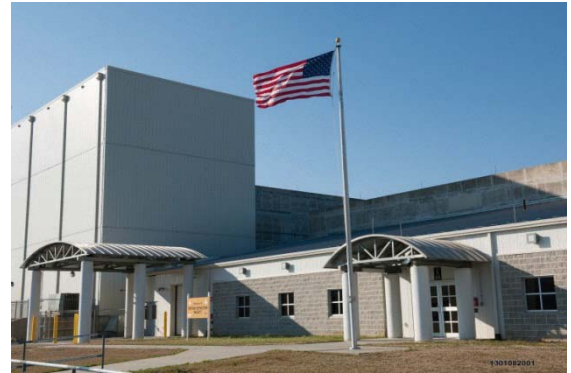
SRS Tritium Extraction Facility
