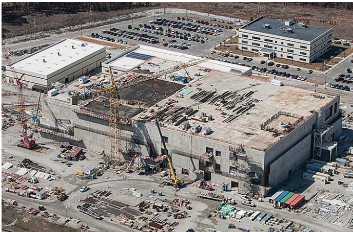
Construction of the Mixed Oxide Fuel Fabrication Facility Progresses
