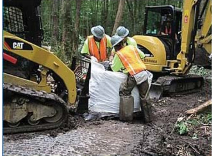
Workers Package Material for Disposal
