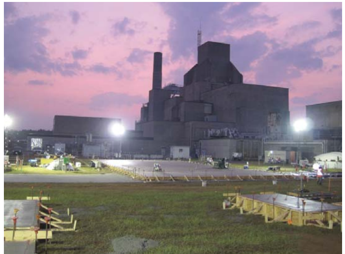
Construction of the Evaporator Building at C Reactor
