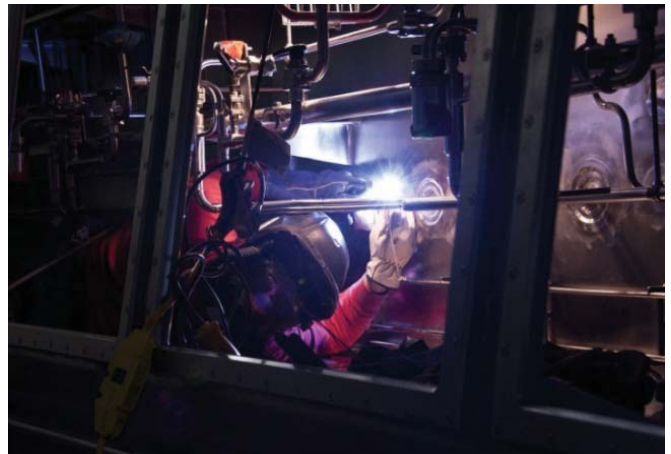
Workers Installing Equipment in the Waste Solidification Building
