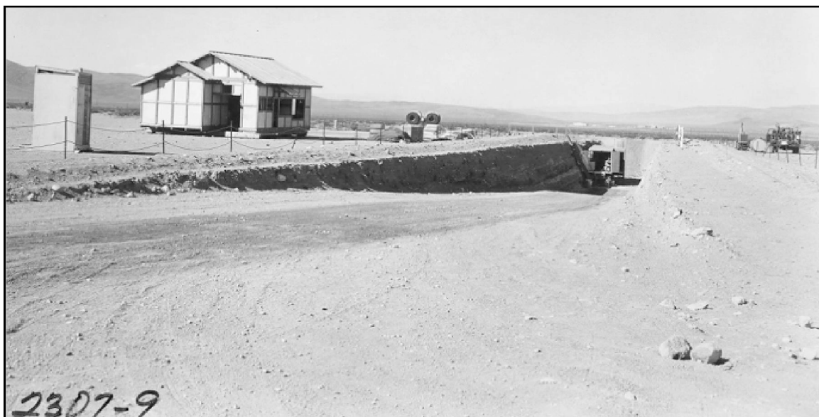
Photo 48. The revetment behind (north) the analog Japanese House held recording trailers for some of the Operation HENRE experimental programs. A metal T-post and rope fence surrounded the revetment. View is to the west. Photo taken September 28, 1966 (Photo 2307-9 on file at NNSA/NSO Nuclear Testing Archive).
