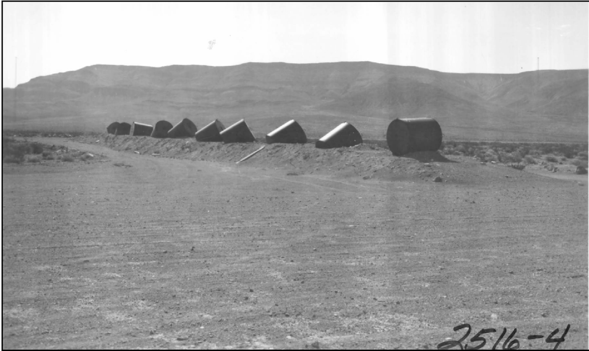
Photo 33. Row of 10 collimators at 1,800 ft from BREN Tower. The raised earth berm and bladed path are clearly visible. Photo taken during Operation HENRE, August 1967. View is east-southeast (Photo 2516-4 on file at NNSA/NSO Nuclear Testing Archive).
