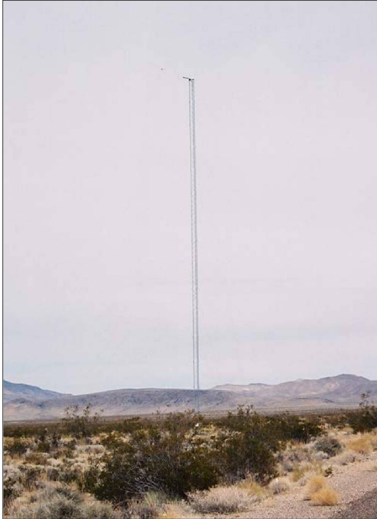
Photo 58. Tower 3.2 used in Operation HENRE Program 3. The pulley and cable system used to suspend the instrumentation for the experiments is visible at the top of the 150 ft tower. View is to the northeast. Photo taken by DRI on November 1, 2006 (on file at NNSA/NSO Curation Facility).
