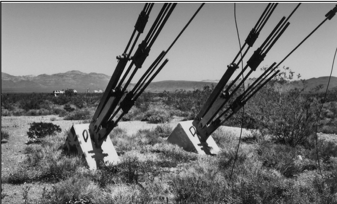
Photo 8. Detail view of one of the six pairs of stanchions that anchor the guy wires stabilizing the 1,527 ft tower. View is to the north-northeast. Photo taken by DRI in June 2004 (on file at NNSA/NSO Curation Facility).
