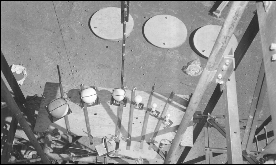
Photo 65. An arc of three cylindrical foxholes used in Operation HENRE Program 5 appear in this photo taken on July 10, 1967 from the main work platform on the BREN Tower. All three have their concrete covers in place as a safety precaution (Photo 2491-3 on file at NNSA/NSO Nuclear Testing Archive).
