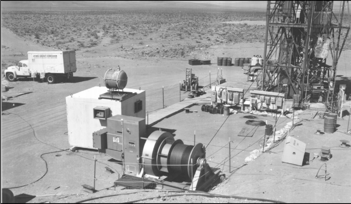
Photo 17. The large winch that lifted the hoist car carrying the Operation HENRE neutron generator assembly is in the center. The brockhouse and wooden walkway to the tower were removed after HENRE ended. The photo was taken from the top of the control bunker on August 18, 1967. View is to the southwest (Photo 2530-13 on file at NNSA/NSO Nuclear Testing Archive).
