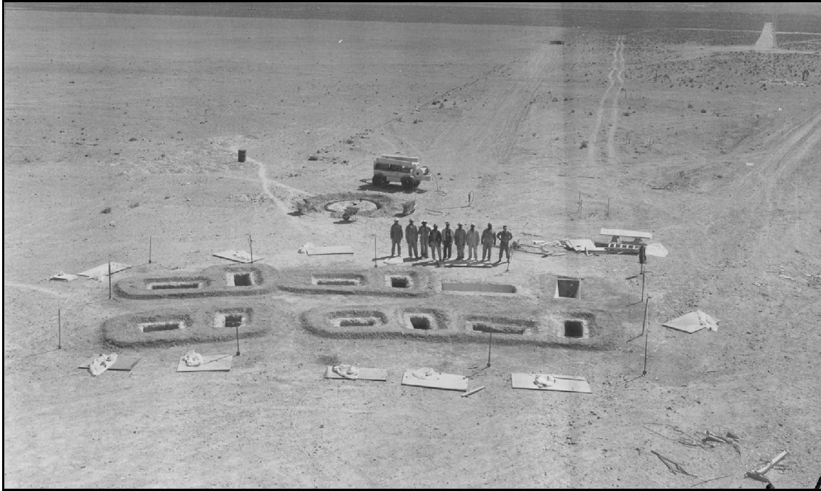
Photo 62. Overview of the rectangular foxholes with plywood covers built for Operation HENRE, Program 3 in 1966. A metal T-post and rope fence surrounds the area. View is to the north (Photo 3020-6 on file at NNSA/NSO Nuclear Testing Archive).
