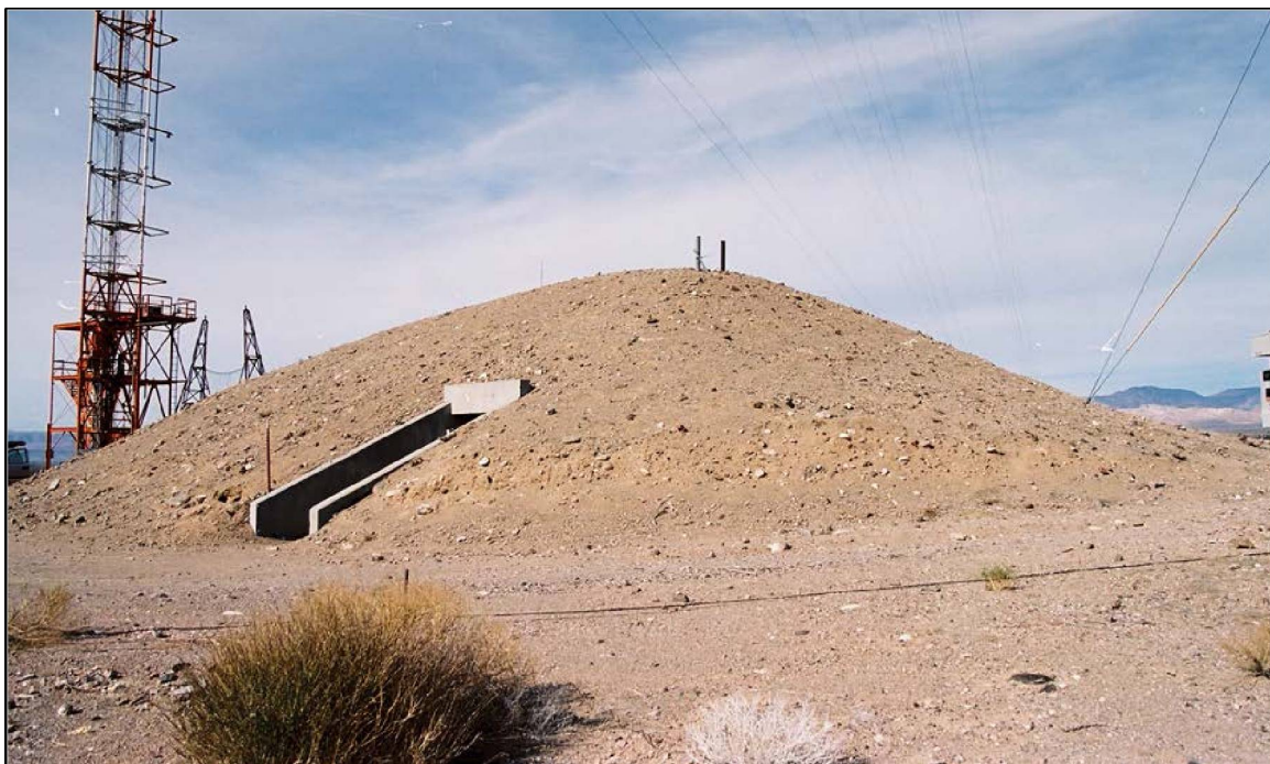
Photo 12. Operation HENRE Control Bunker. BREN Tower and the upper portion of one of the paired 27 ft towers from the 1990s experimental program are visible behind the bunker to the left. View is to the northwest. Photo taken by DRI on November 1, 2006 (on on file at NNSA/NSO Curation Facility).
