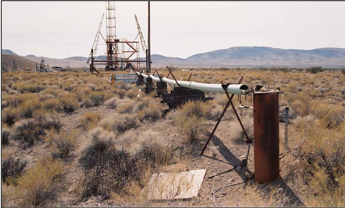
Photo 23. Cable trough leading from the underground civil defense shelter ventilation pipe toward the Control Bunker. View is to the south-southwest. Photo taken by DRI on November 1, 2006 (on file at NNSA/NSO Curation Facility).
