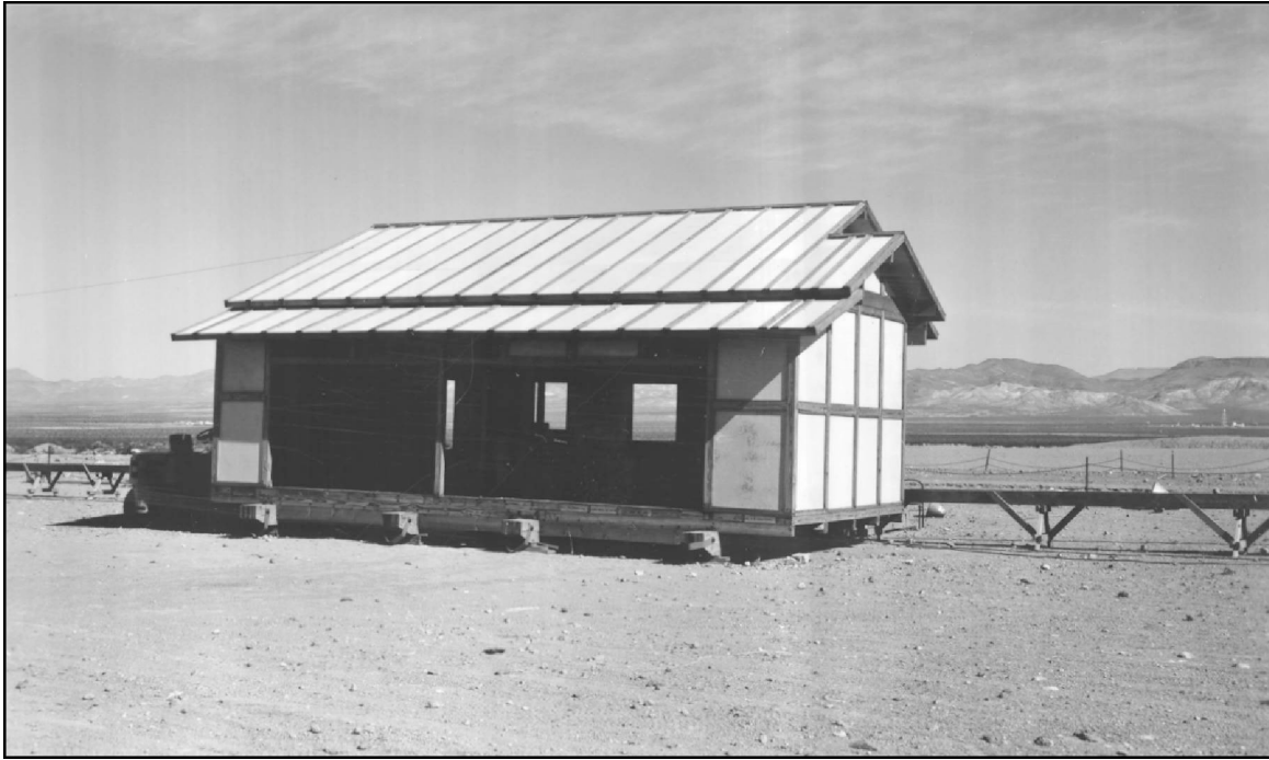
Photo 41. South and east elevations of the analog Japanese House in 1967. Wooden cable troughs for the dosimetry instrumentation are visible on both sides of the house. The fence surrounding the trailer revetment is in the background. View is to the northwest (Photo 2515-14 on file at NNSA/NSO Nuclear Testing Archive).
