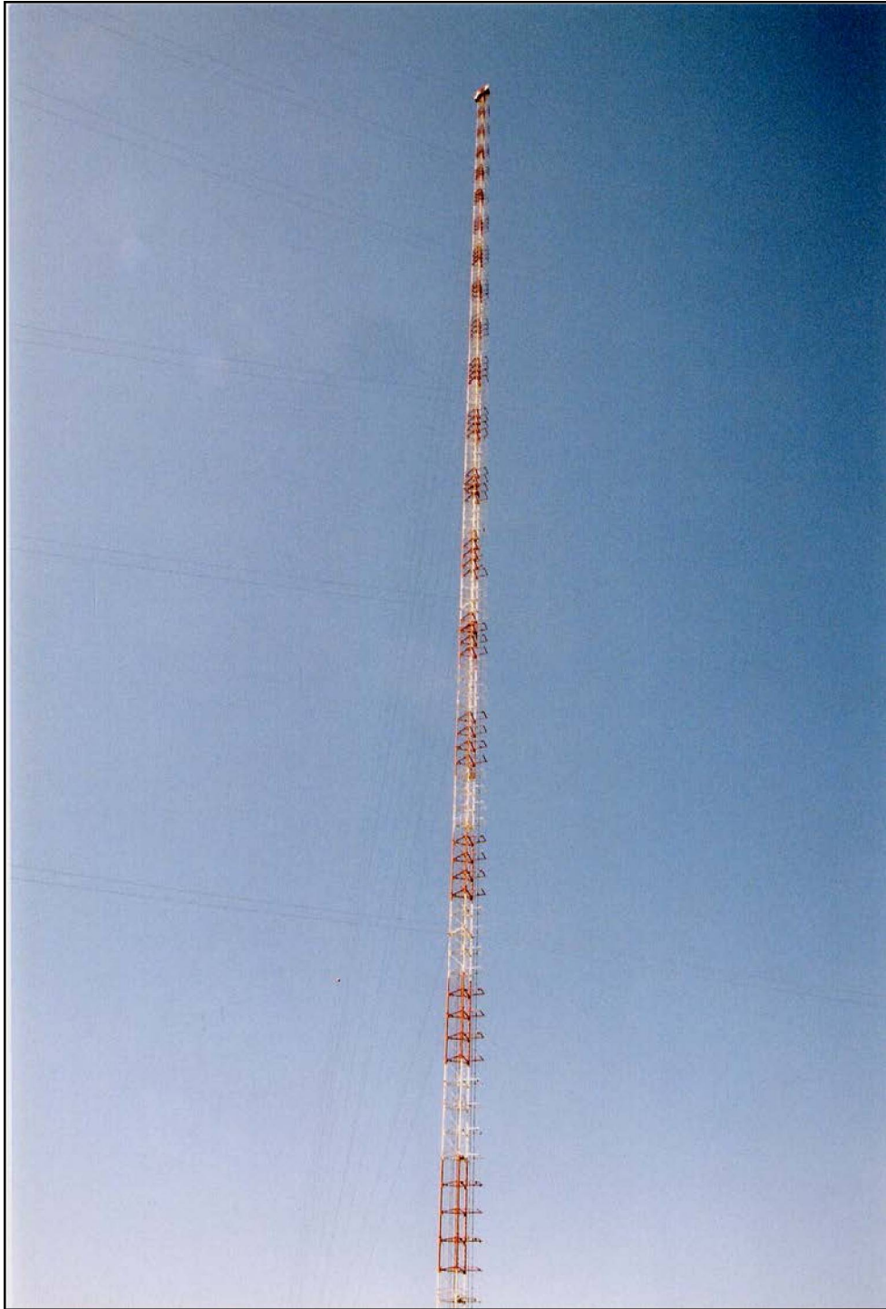
Photo 6. The upper 1,100 ft of BREN Tower in June 2004. Thirty-seven of its fifty-one 30 ft sections are visible. The faint gray lines extending from the tower are the guy wire cables that stabilize the tower. View west-southwest (on file at NNSA/NSO Curation Facility).
