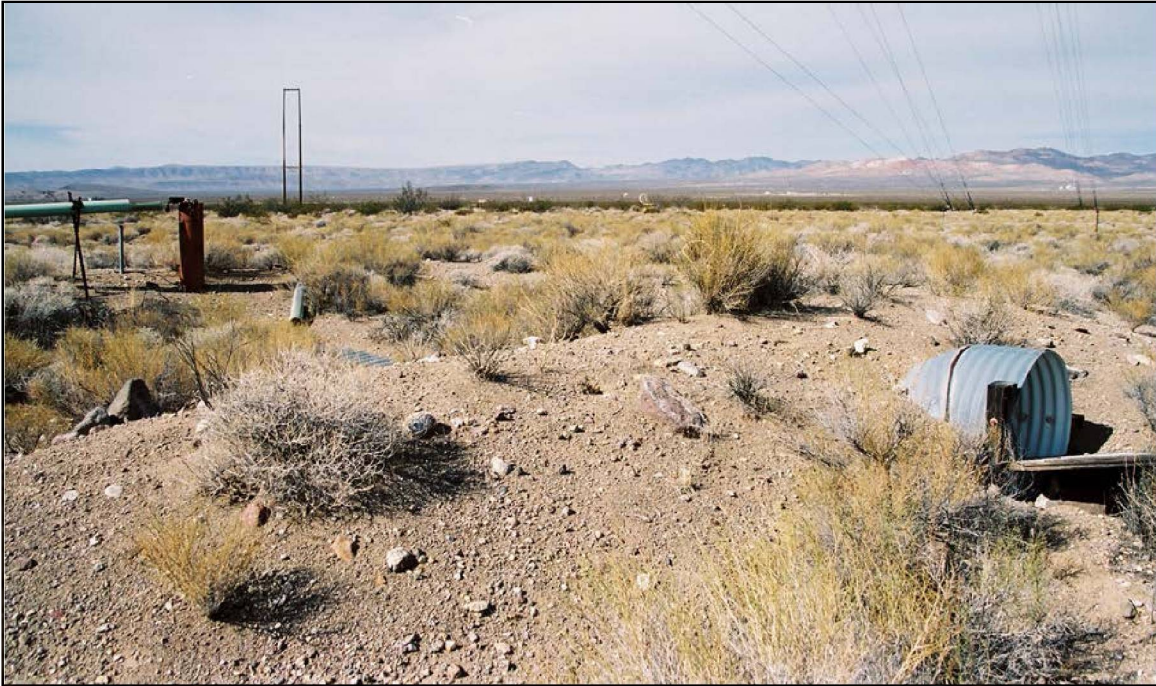
Photo 21. The underground civil defense shelter (aka pipe shelter) was one of the Operation HENRE Program 1 experiments. The shelter extends from the entrance on the right towards the upright ventilation pipe on the left. View to northeast. Photo taken by DRI on November 1, 2006 (on file at NNSA/NSO Curation Facility).
