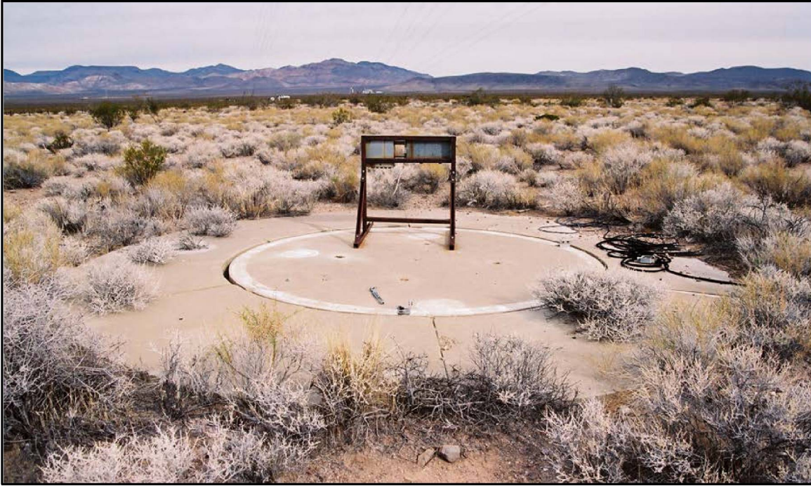
Photo 71. The concrete turntable used for Operation HENRE Program 9 involving shielding studies for the radiological armored pod or RAP. View is to the north. Photo taken by DRI on November 1, 2006 (on file at NNSA/NSO Curation Facility).
