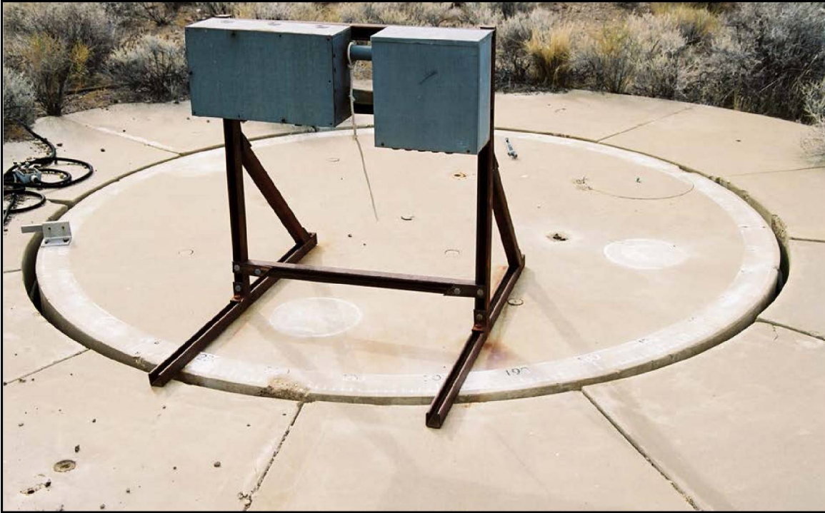
Photo 72. Program 9 equipment and instrumentation were mounted to the turntable stand shown here and rotated into various positions relative to the neutron accelerator mounted on BREN Tower. View to the southeast. Photo taken by DRI on November 1, 2006 (on file at NNSA/NSO Curation Facility).
