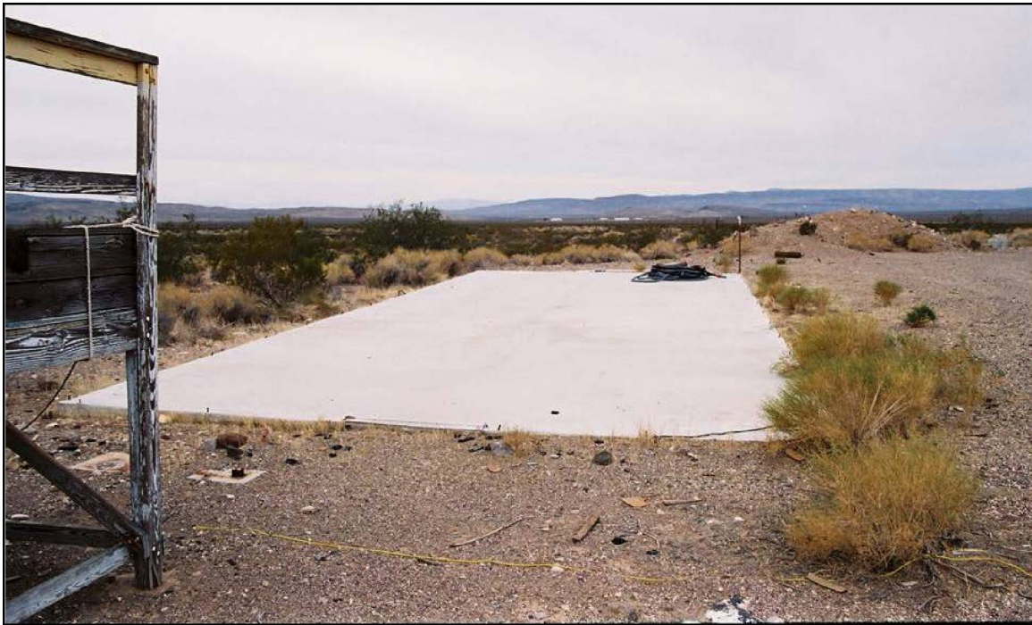
Photo 16. All that remains of the Quonset hut erected during Operation HENRE is the concrete foundation slab. View is west-southwest. Photo taken by DRI on November 1, 2006 (on file at NNSA/NSO Curation Facility).
