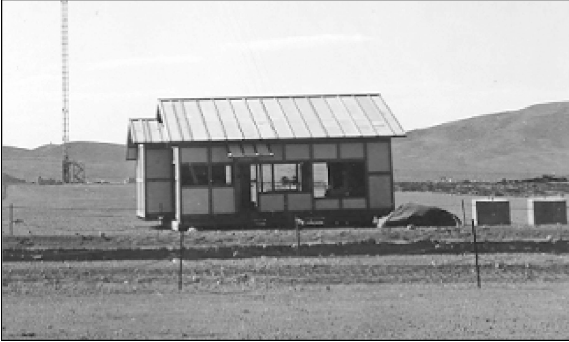
Photo 39. North elevation of the analog Japanese House in 1967. The fenced instrument trailer revetment is visible in the foreground and the two concrete prisms used in the dosimetry studies sit to the right (west) of the house. View is to the south (Photo 2307-8 on file at NNSA/NSO Nuclear Testing Archive).
