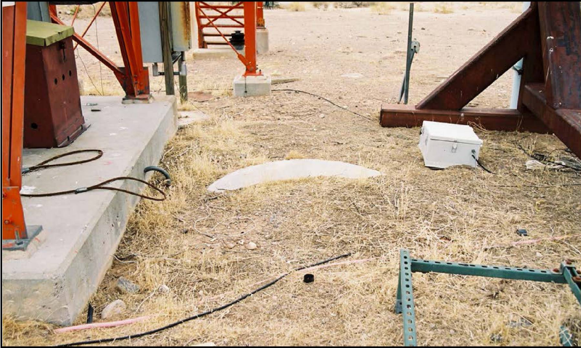
Photo 67. The Program 5 cylindrical foxhole located at the base of BREN Tower is almost completely covered with earth. Only a portion of the concrete cover is visible. View is to the west. Photo taken by DRI on November 1, 2006 (on file at NNSA/NSO Curation Facility).
