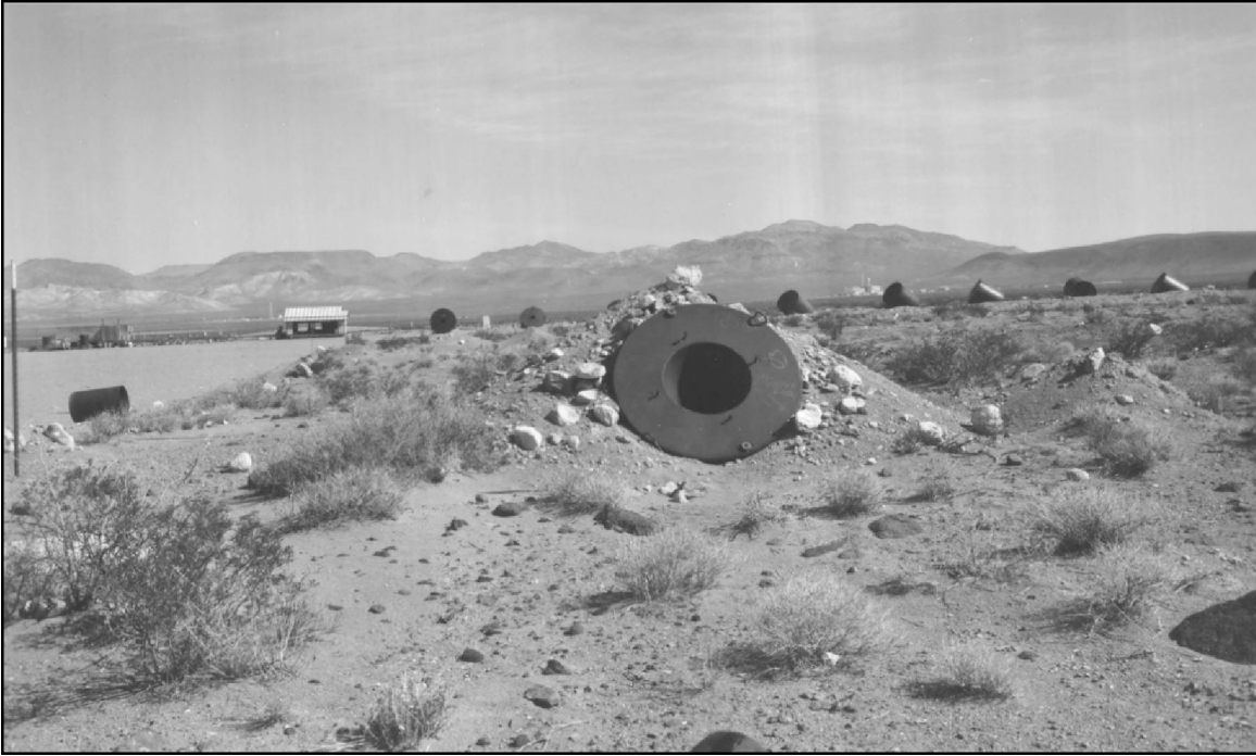
Photo 29. August 1967 photograph of the eastern member of a pair of partially buried collimators located 1,520 ft from BREN Tower. (Photo 2516-10 on file at NNSA/NSO Nuclear Testing Archive).
