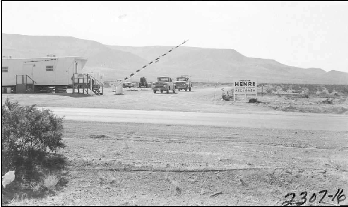
Photo 78. The gated entrance to the BREN Tower Complex in Area 25, September 28, 1966. Cane Spring Road runs across the photo. View is to the southeast (Photo 2307-16 on file at NNSA/NSO Nuclear Testing Archive).
