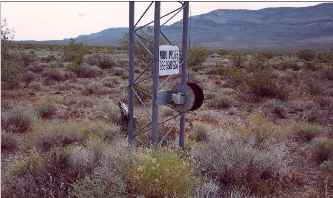
Photo 60. The hand-cranked winch on the base of Tower 3.2. The placard identifies the tower as part of the NDRL Operation HENRE Experimental Program 3 and provides contact phone numbers. View is to the southeast. Photo taken by DRI in June 2004 (on file at NNSA/NSO Curation Facility).
