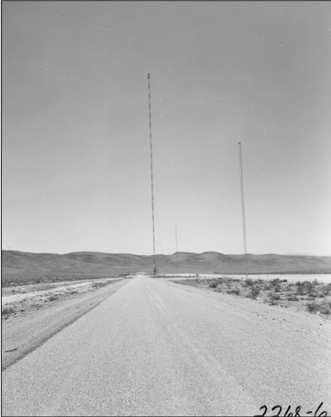
Photo 56. The BREN Tower (center of frame) dwarfs the three 150 ft towers used for Operation HENRE Program 3. During the neutron accelerator runs, instruments were suspended from cables strung between the towers 120 ft above the ground. Photo taken from the paved access road on July 1, 1966. View is to the southwest (Photo 2268-6 on file at NNSA/NSO Nuclear Testing Archive).
