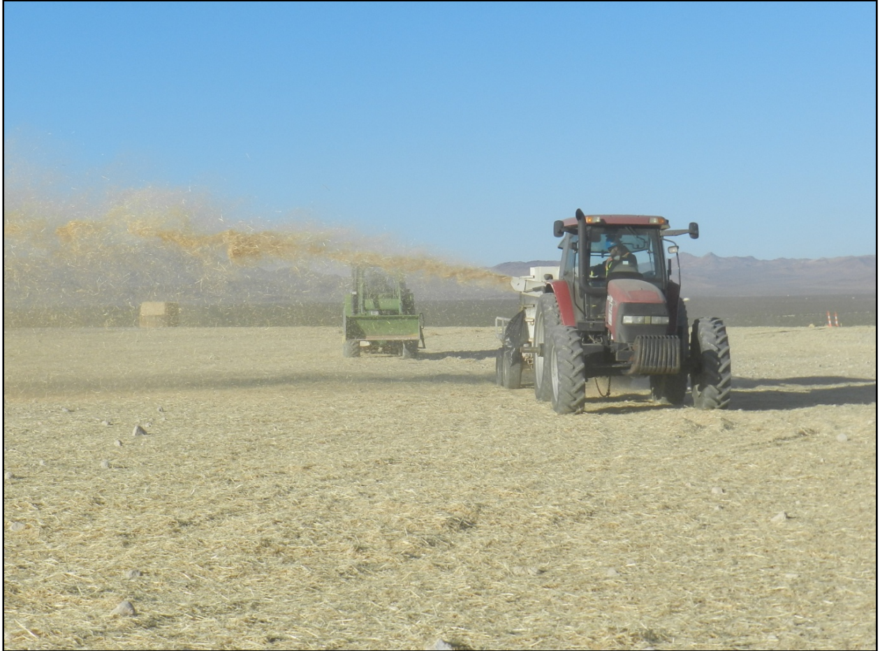
Figure 7-4. Straw mulcher followed by tractor with Finn crimper used to secure the blown straw (Photo by D. Anderson, November 9, 2011)
