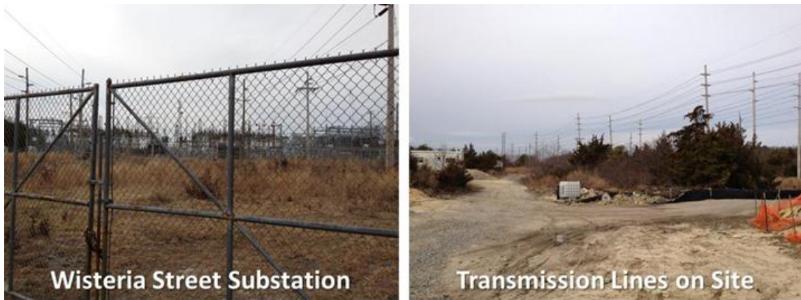
Figure 9. Wisteria Street Substation and electrical transmission lines at the Price Landfill. Photos by James Salasovich, NREL
