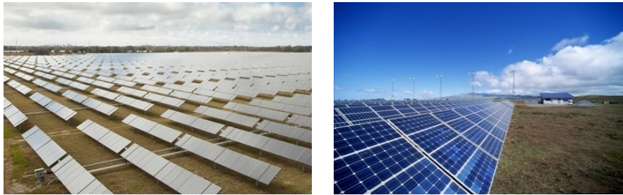
Figure 3. Mono- and multi-crystalline solar panels. Photos by (left) SunPower Corporation, NREL 23816 and (right) SunPower, NREL 13823
