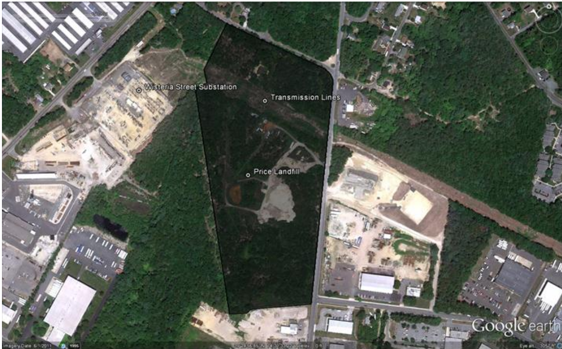
Figure 8. Price Landfill, transmission lines, and the Wisteria Street Substation
