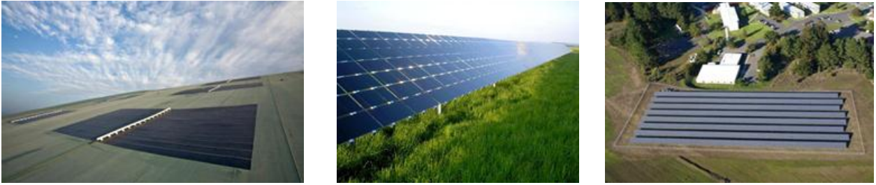
Figure 4. Thin-film solar panels installed on (left) solar energy cover and (middle/right) fixed-tilt mounting system. Photos by (left) Republic Services, Inc., 23817; (middle) Beck Energy, NREL 14726; and (right) U.S. Coast Guard Petaluma site, NREL 17395
