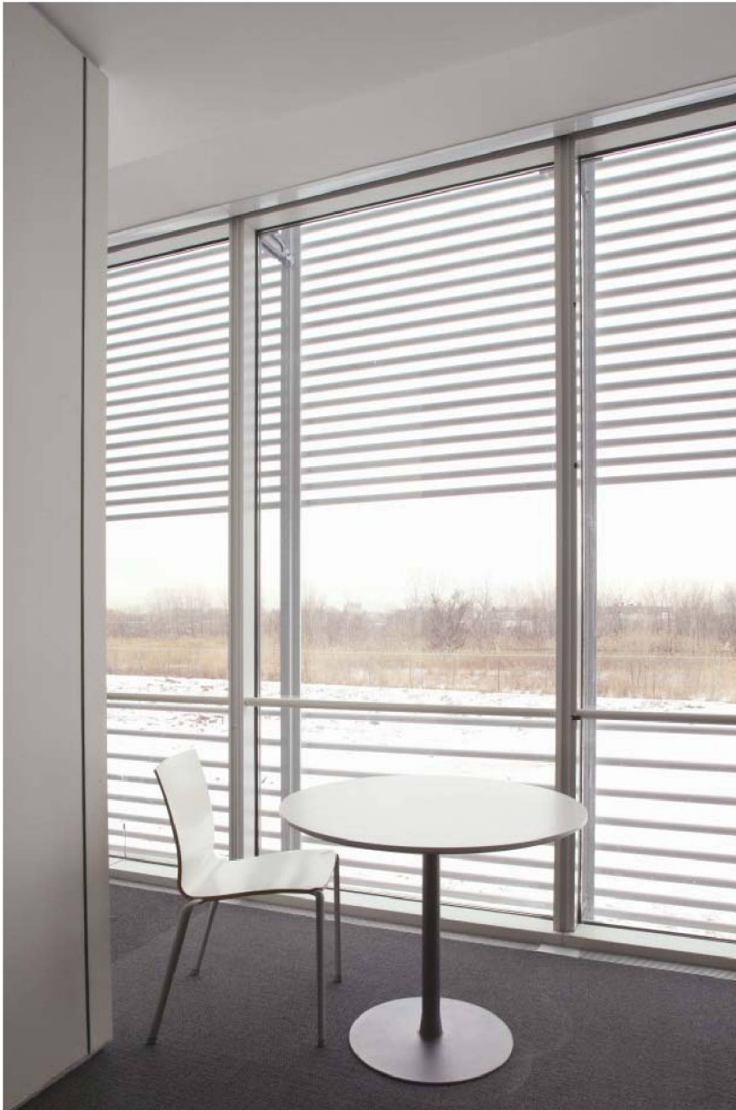
Figure 5. The view section of the window wall is the open portion between the upper and lower exterior shading elements (photo from the daylighting mockup at College Point, New York). Copyright: LBNL.
