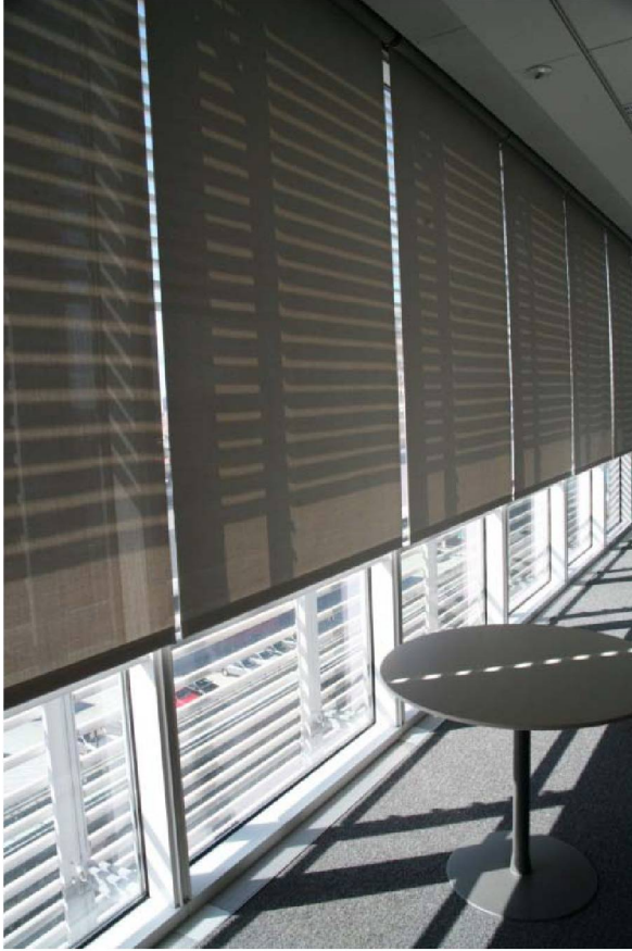
Figure 13. The automated shades controlled direct sun to within 3 ft from the window wall at floor level in most open plan work areas. Copyright: LBNL.
