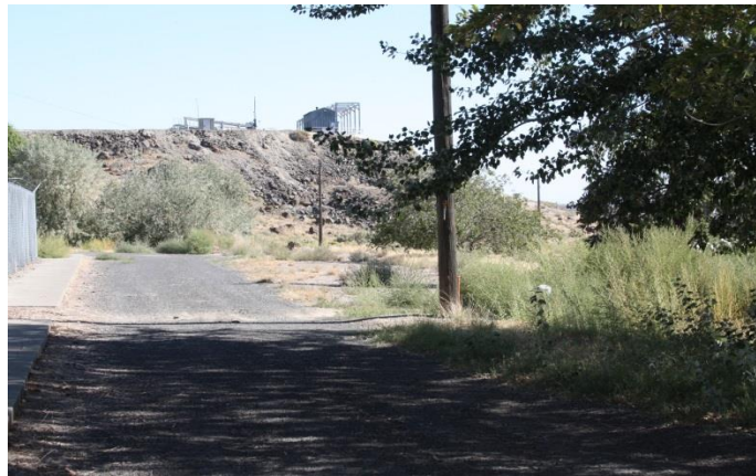
Figure A.4. Potential background air monitoring location – Yakima Valley area Chandler Power Plant Irrigation Pump Station (middle) looking E toward upper
