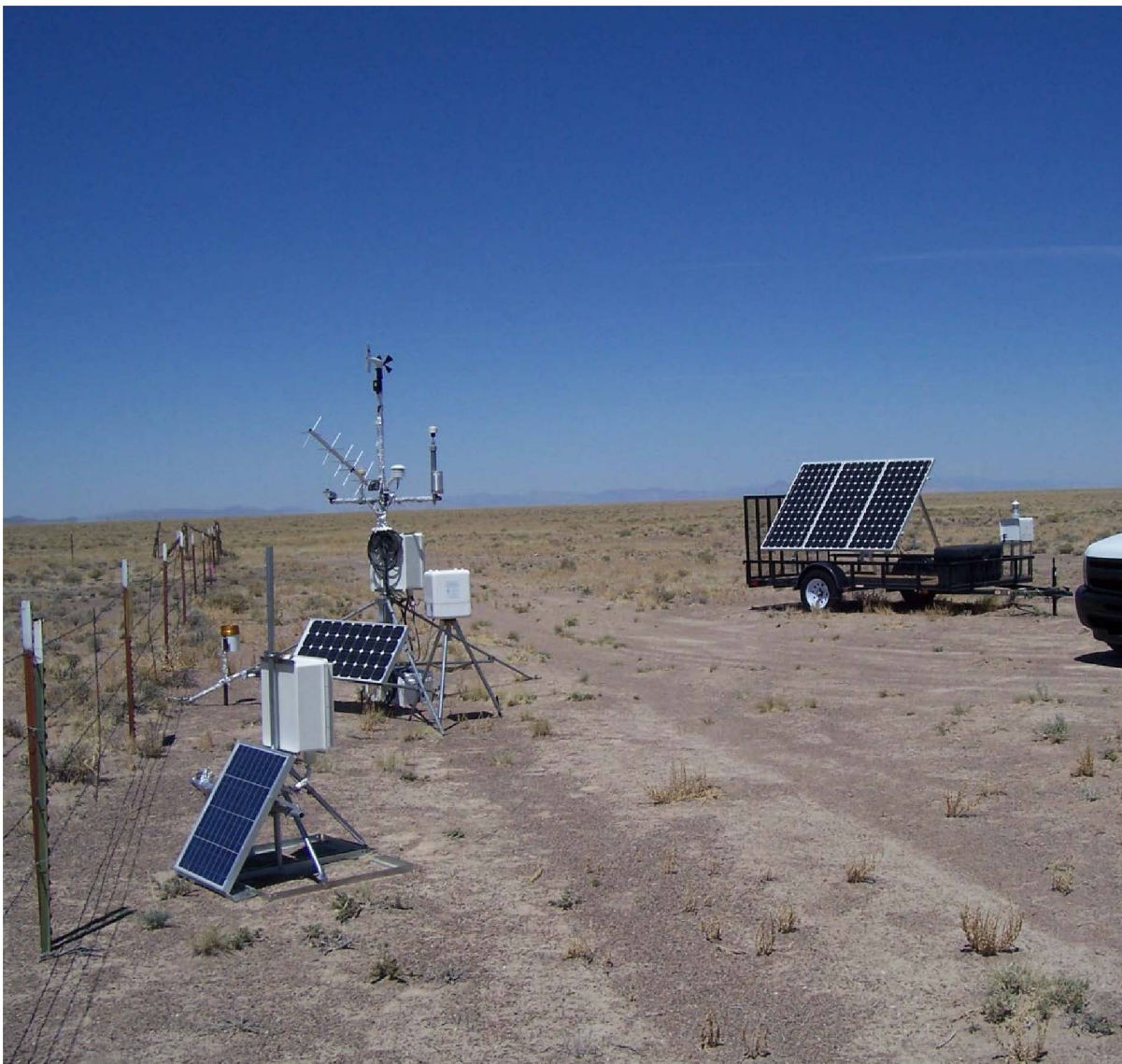
Figure 5. The solar powered air sampler, saltation sensor, and meteorological tower (center right, foreground left, and center left, respectively) at Station 402 are located along the north fence that bounds the Clean Slate I contamination area.
