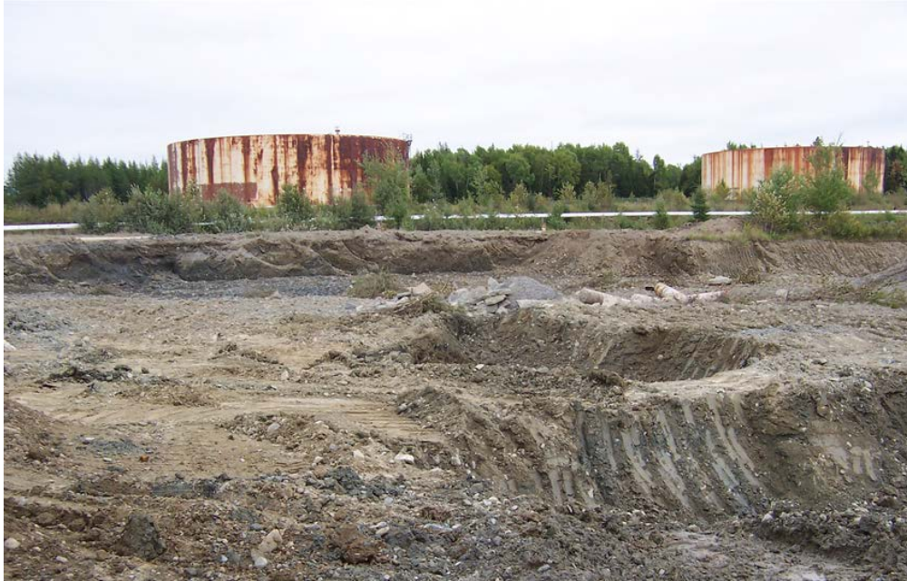
Figure 3. Tanks at Loring site. Photo from Mike Daly, EPA
