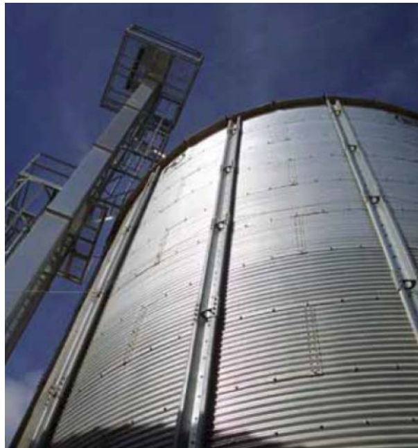
Figure 28. Pellet storage silo
