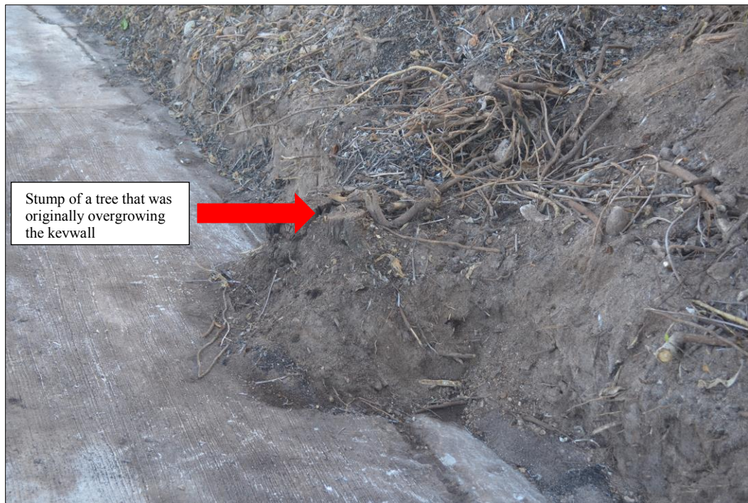
Fig 14. A photo of a tree stump located over the keywall (the stump was later removed) (Visual Survey, May 2013).
