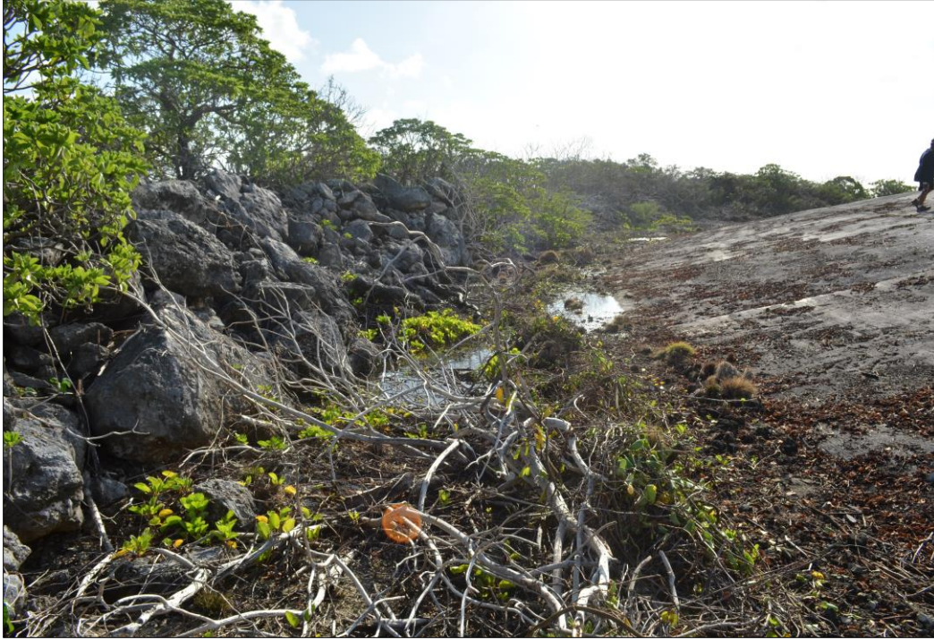
Fig. 4a. Vegetation growing on the inside of the riprap 'mole wall' surrounding the Cactus crater containment structure on Runit Island (Visual Survey, May 2013).
