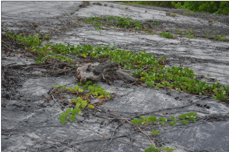
Fig 12. Vegetation growth over the face of Runit Dome (Initial conditions, Visual Survey, May 2013).
