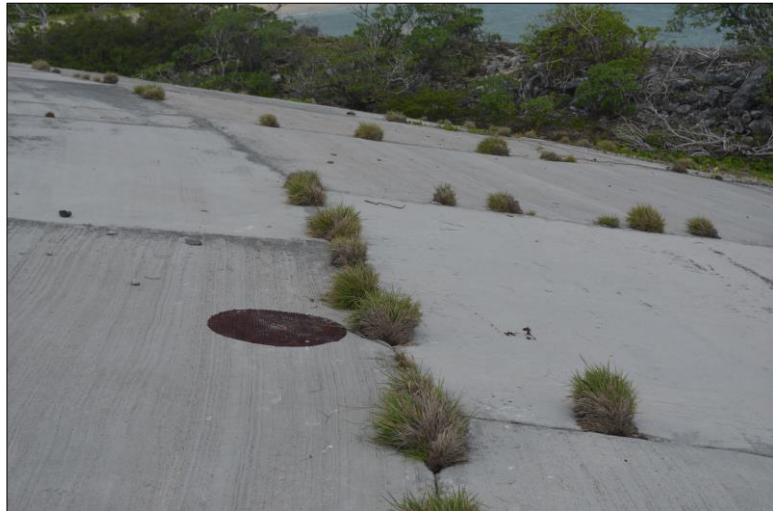
Fig 12. Vegetation growth over the face of Runit Dome (Initial conditions, Visual Survey, May 2013).
