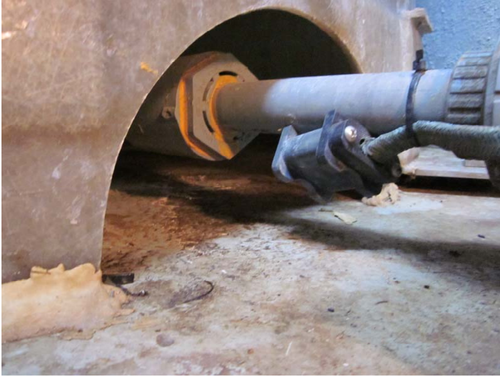
Figure 4. Access for Installed Camera to View the Area under the Tank
