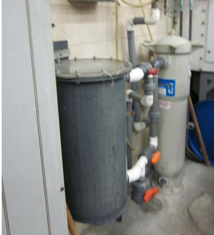
Figure 8. Canister On the Left Contains a Stainless Steel Basket; Canister On The Right Contains a 50 Micron Filter Sock. Drain on the Floor Discharges into the Secondary Containment.
