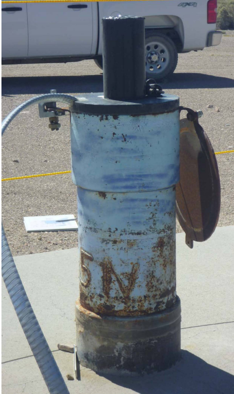
Figure 24. UE-5n wellhead, view to the south.
