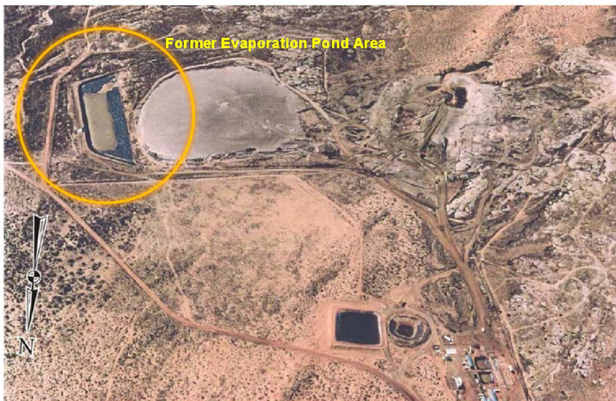
Figure 3. Evaporation Pond at the Monument Valley Site During Milling Operation (March 1993) Photo is from the 2010 assessment (DOE 2010). Note orientation of north arrow.
