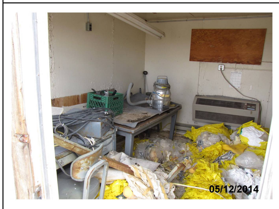
Figure F.1-1 Photographs of Wood Shed at CSII
