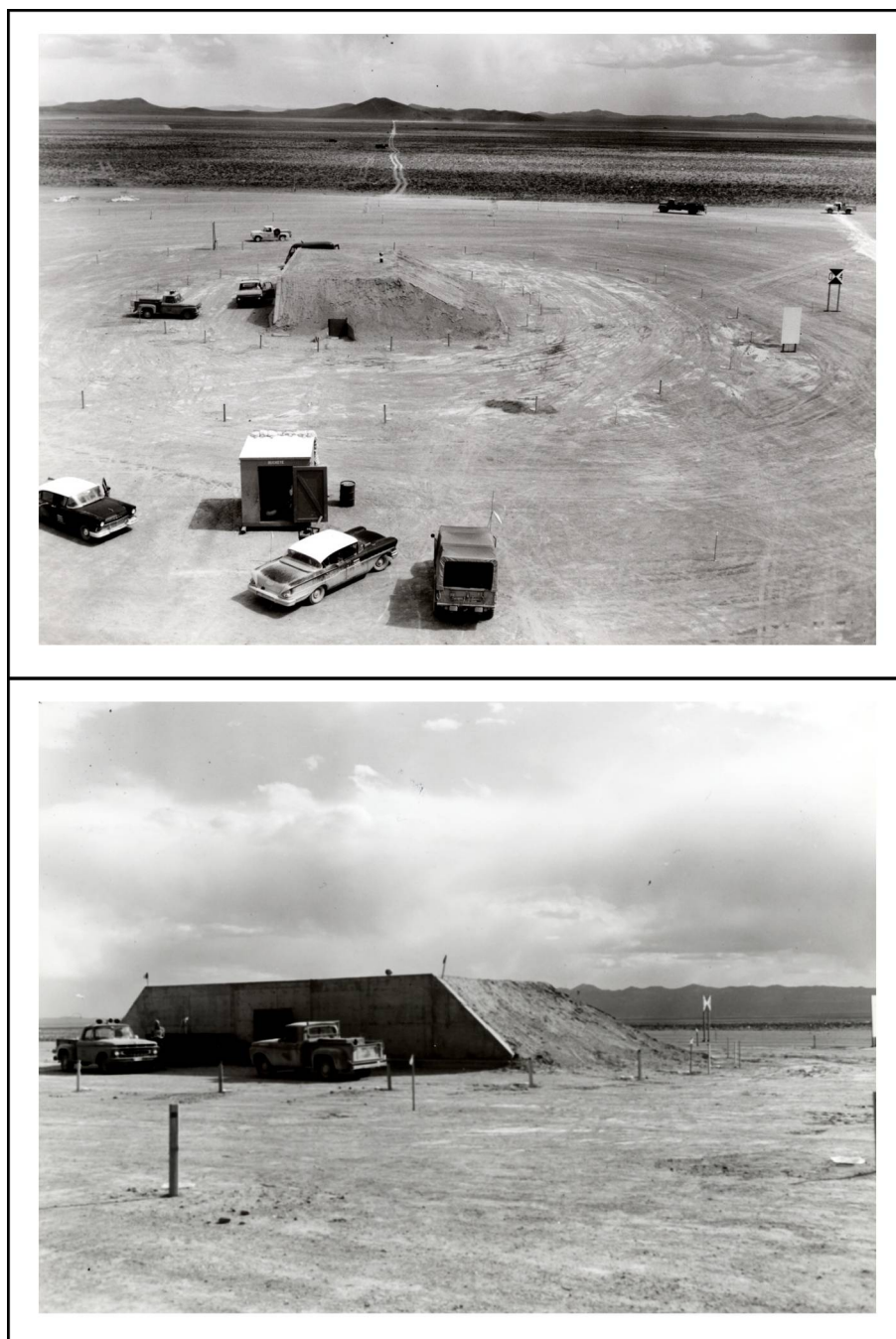
Figure 2-6 Pre-test Photographs of the CSII Structure (1963) Source: NNSA/NSO, 2004
