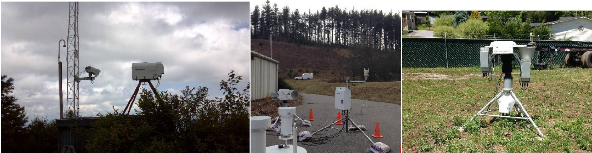
Figure 1. Left to right: MWR2C, eastern MWR3C, and inner region valley MWR3C.
